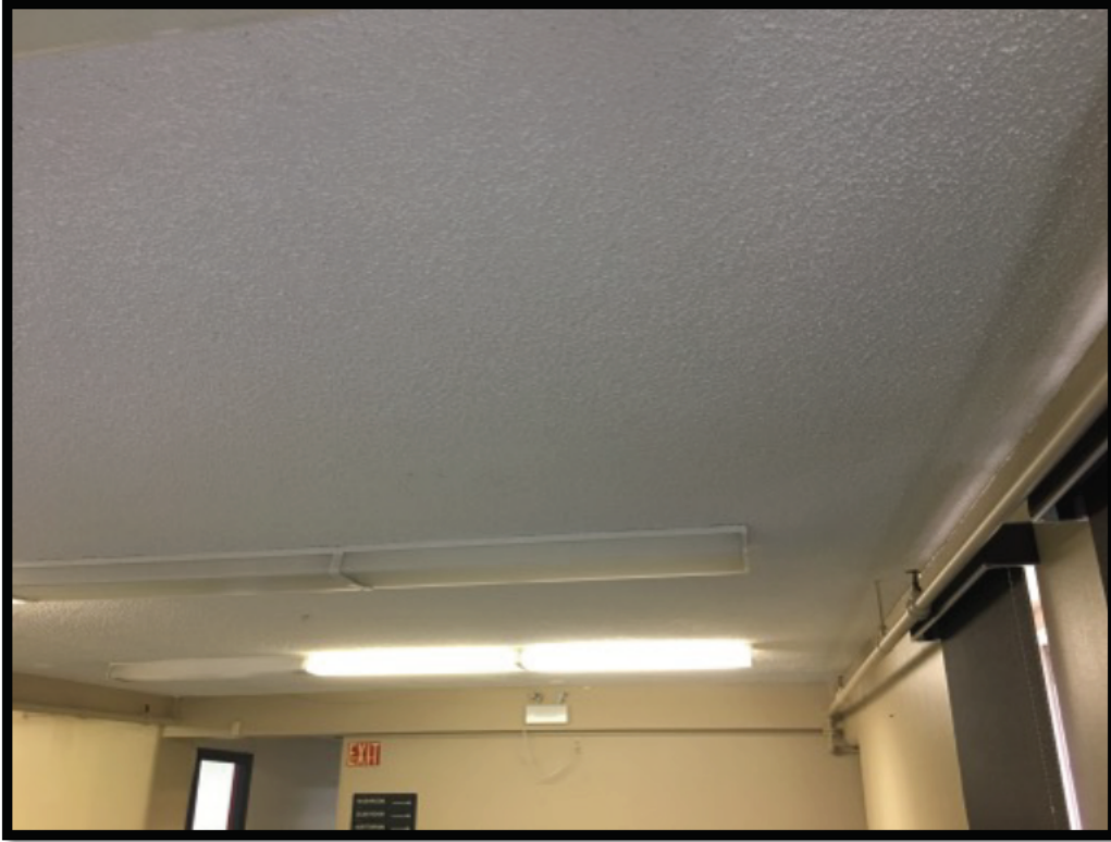
Sample A5 – Ceiling Texture / Main Floor Lobby
