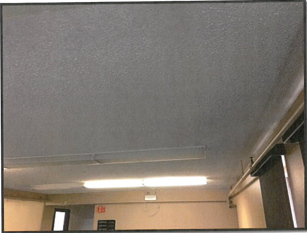
Sample A5 – Ceiling Texture / Main Floor Lobby
