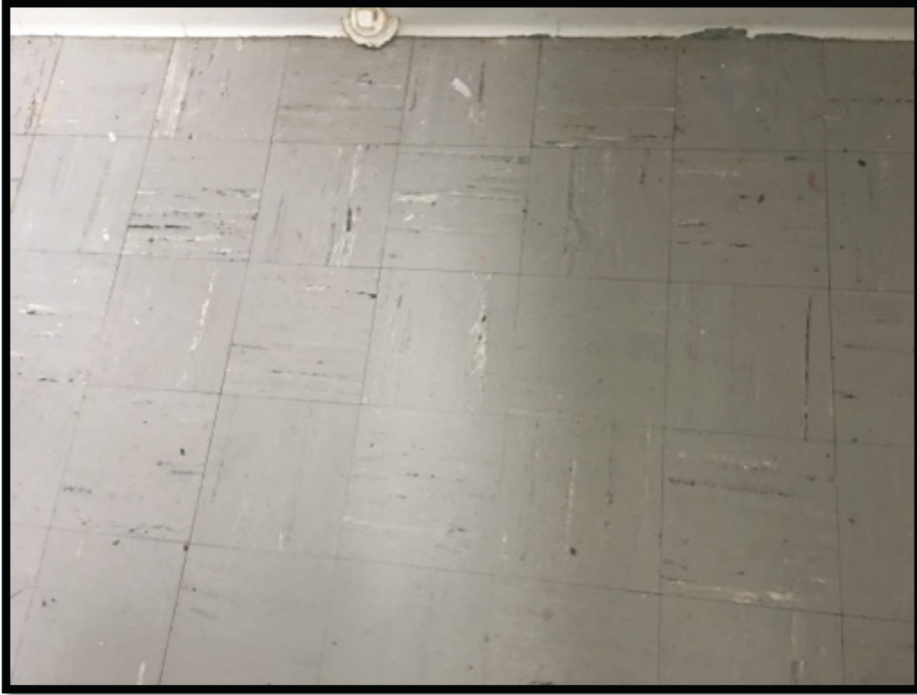
Sample A9 – Blue Floor Tile / Main Women’s Washroom
