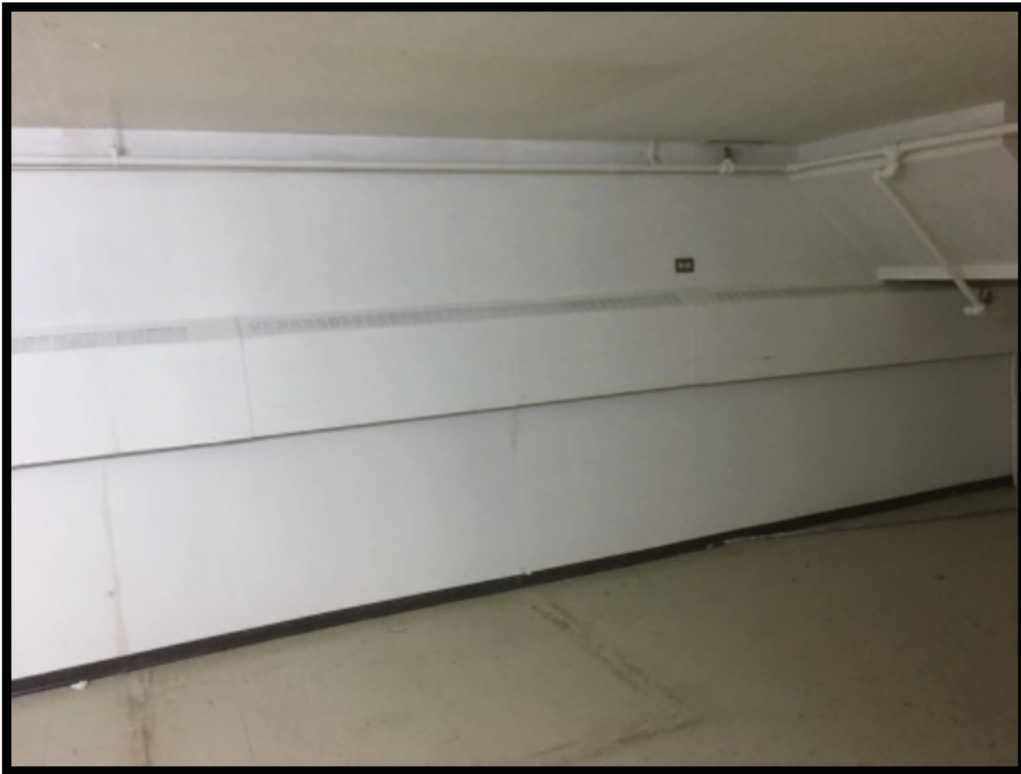
Sample A23 – Joint Compound; Walls & Ceiling/ Auditorium Storage Rm
