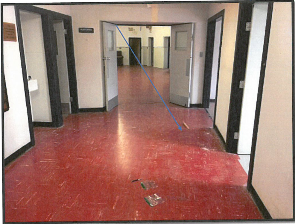
Sample A7 – Red Floor Tile/ Auditorium Entrance
