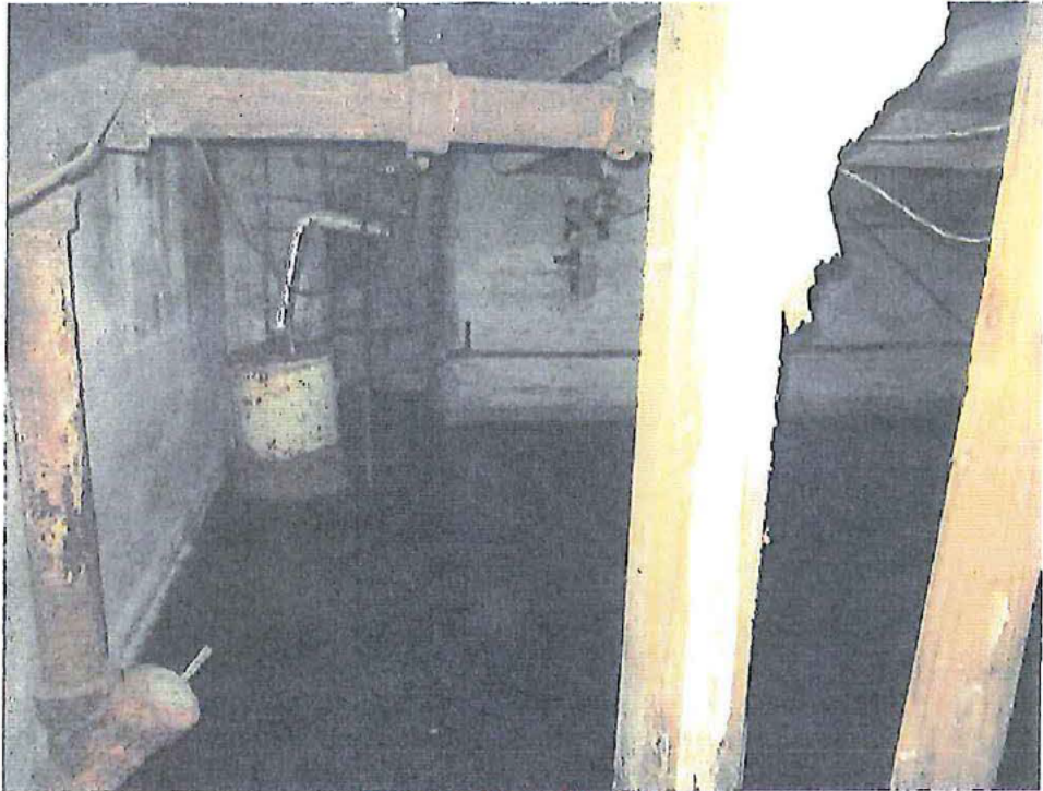
Picture 1 - Flooded Basement
