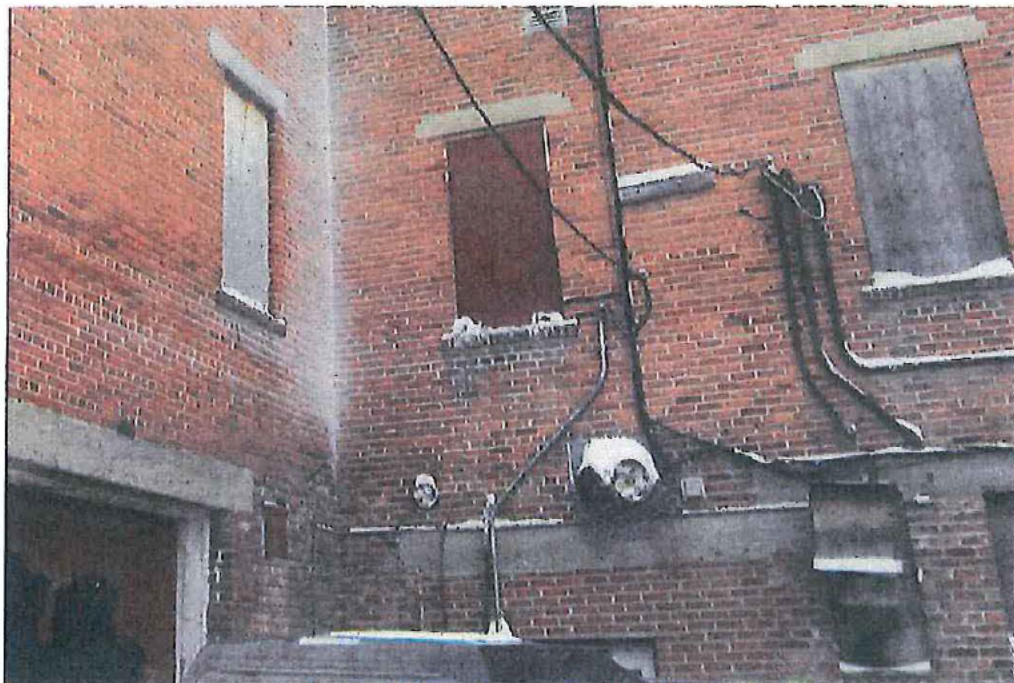
Picture 6 - Deteriorated brick along East
