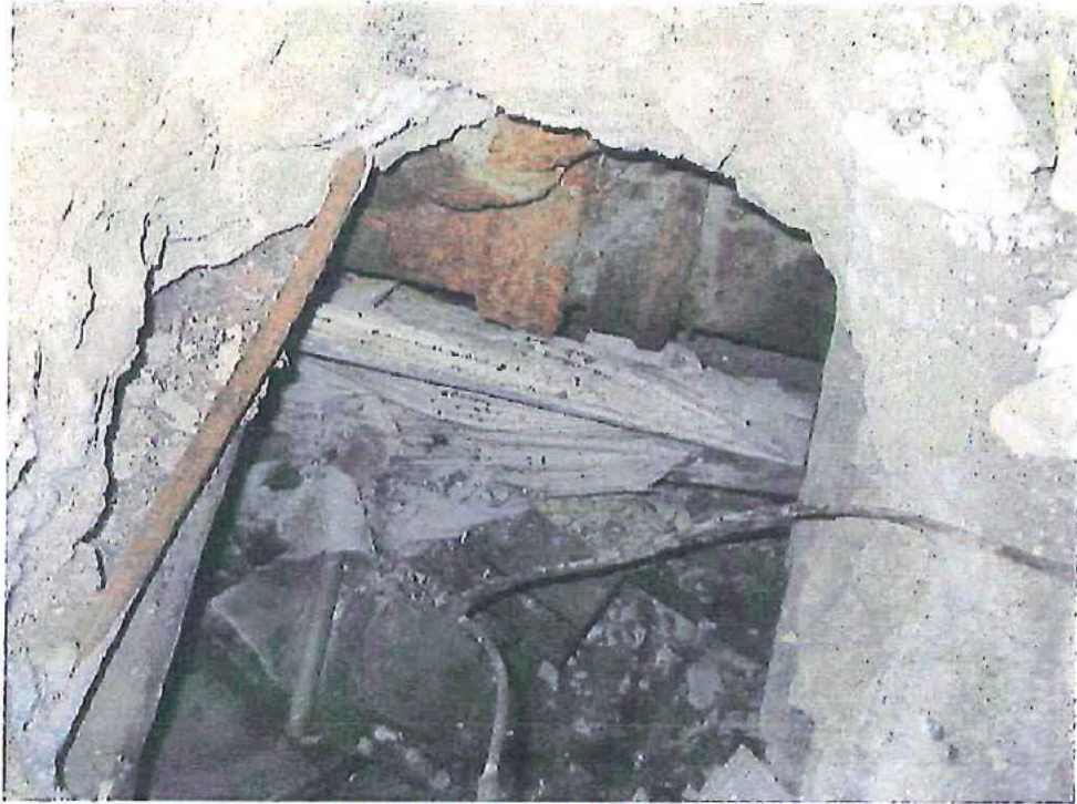
Picture 3 Mechanical duct under slab
