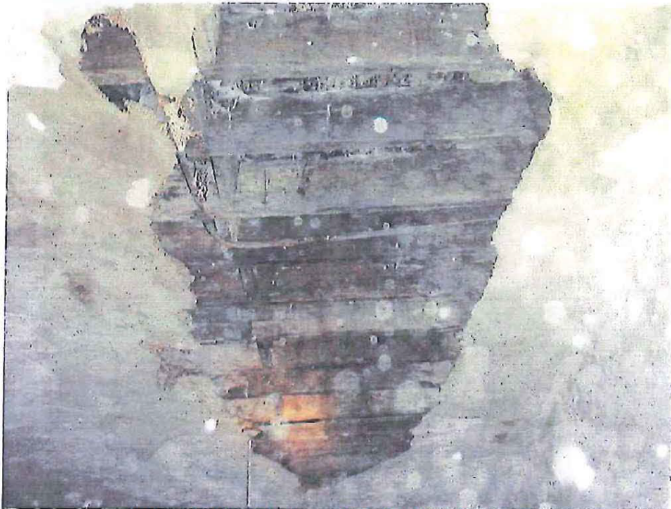
Picture 4 – Water damaged and deteriorated 2nd floor joists
