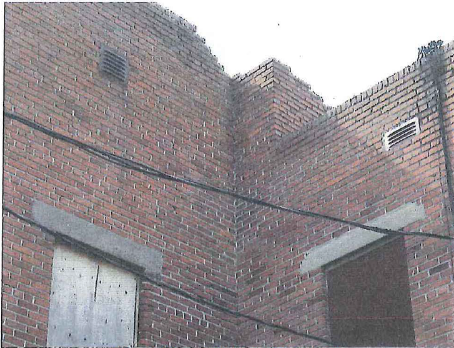
Picture 5 - Removed or fallen-parapet brick work
