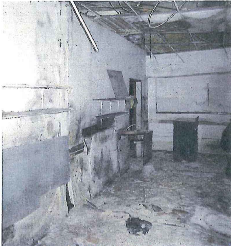
Picture 2 - finishes throughout main floor
