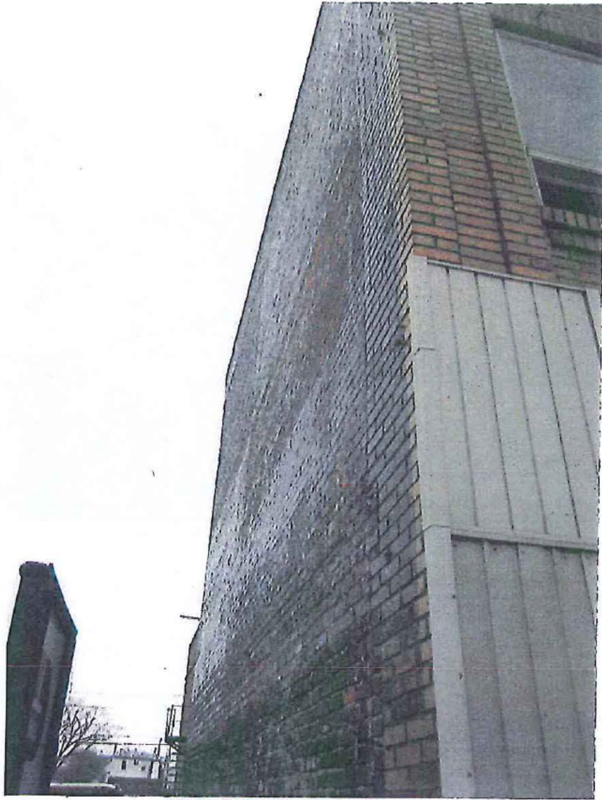
Picture 7— Leaning North brick wall
