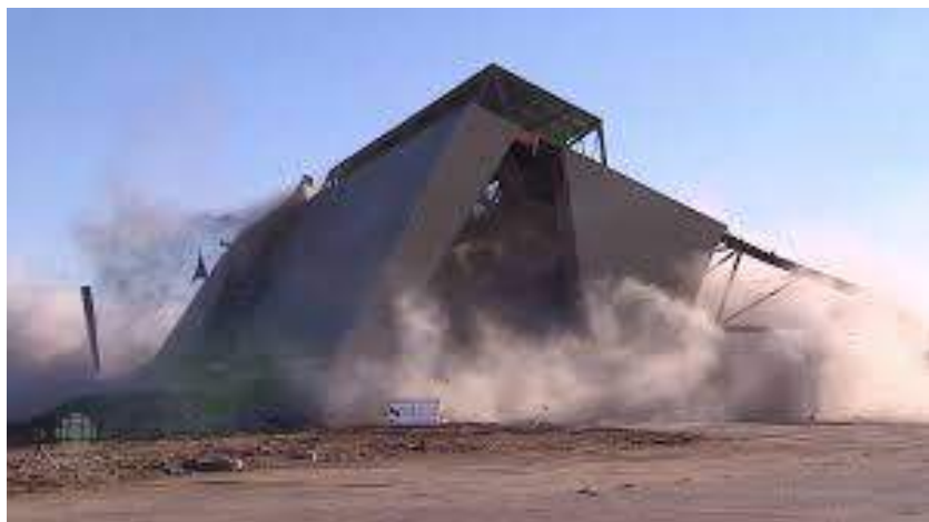
Figure 2: The controlled collapse of the west grandstand at Taylor Field.
