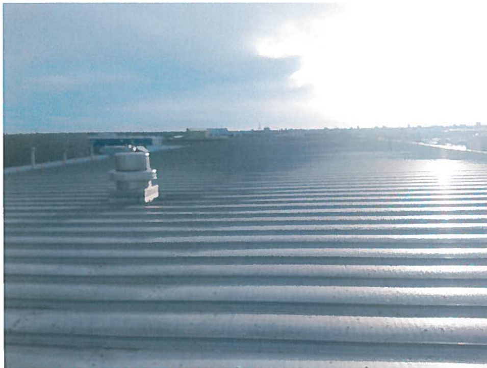
Roof – 1993 Structure looking South
