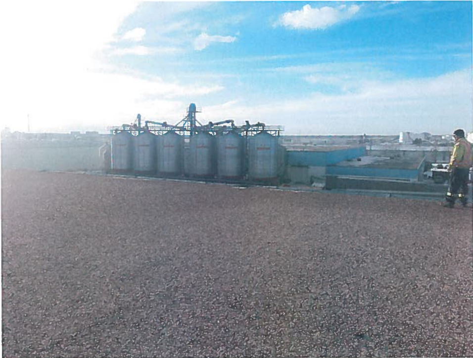
Roof – Original Structure looking South West
