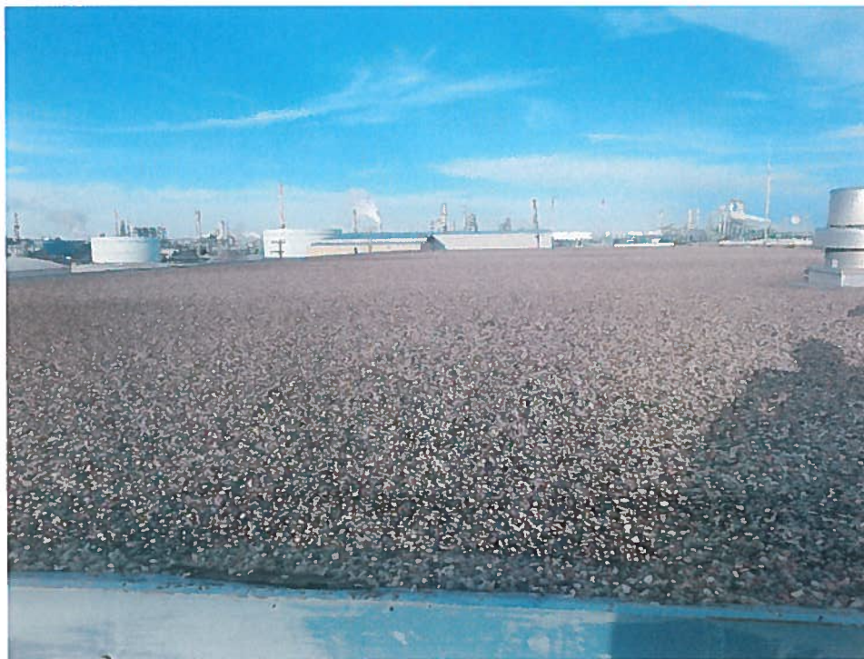
Roof – 1988 Structure looking North
