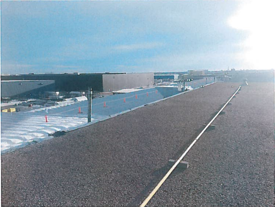
Roof – Original Structure looking South east
