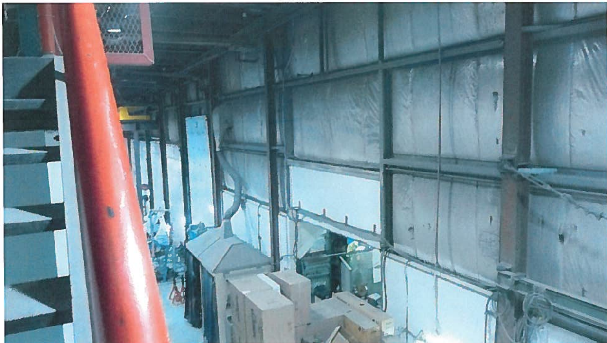
Main Floor – Manufacturing Area
