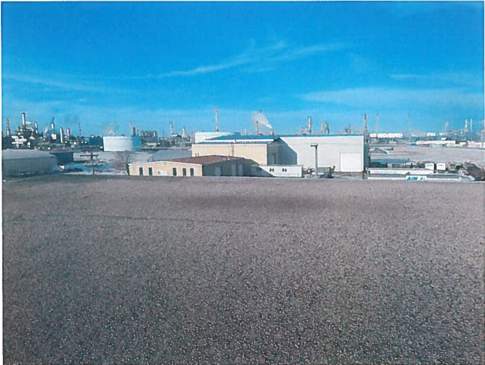
Roof – Original Structure looking North
