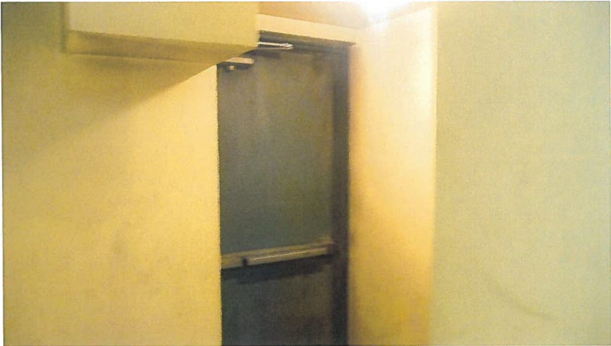
2 nd Floor finished mezzanine – Far end of lunch & locker room – Egress
