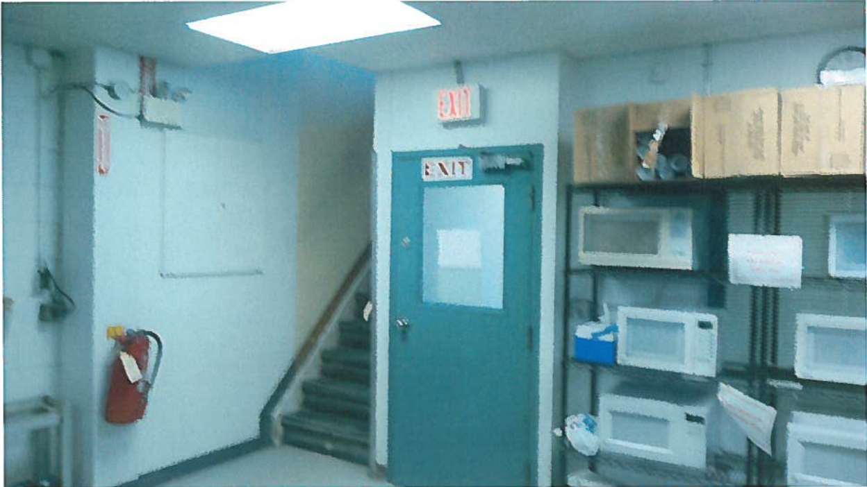
Main floor lunch and locker room – Staircase to 2 nd level finished mezzanine
