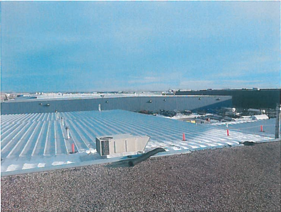
Roof – Original Structure looking East
