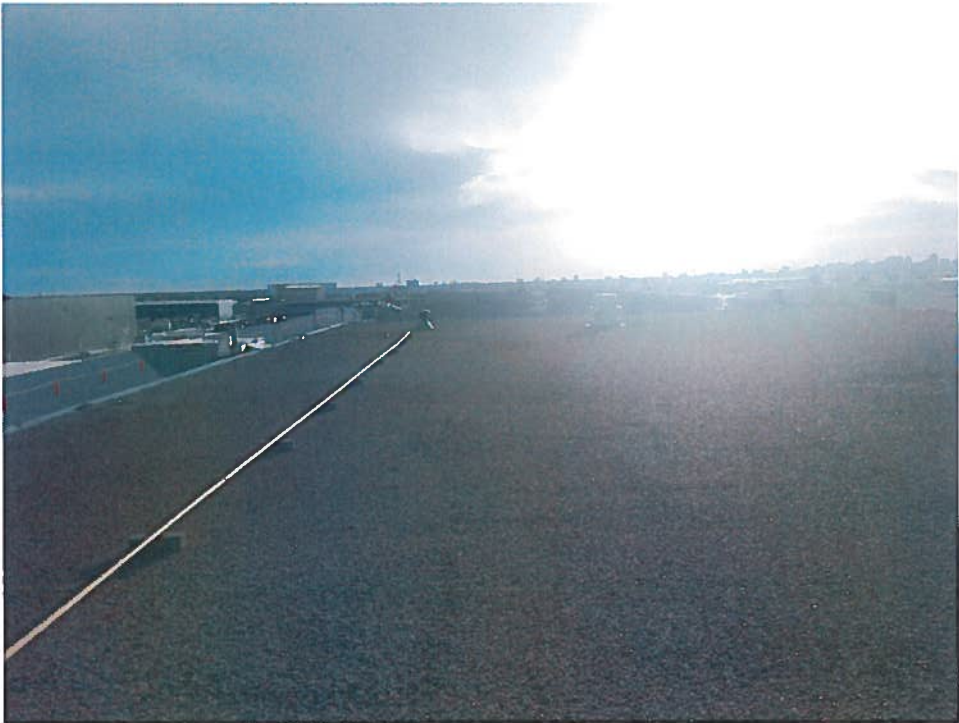
Roof – Original Structure looking south
