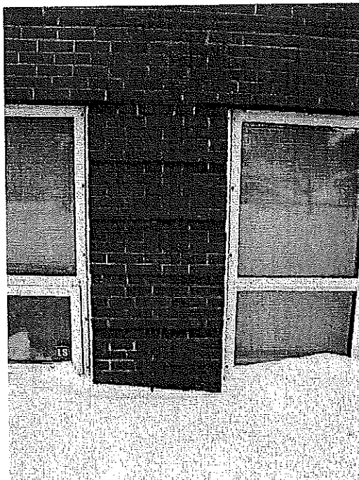
Figure 9 — running bond on steel lintels (replaced brick arch lintel)
