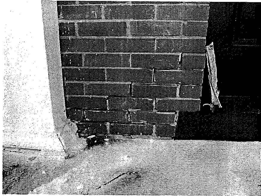
Figure 14 – Damaged masonry at both sides of the main entrance doors at top of stairs
