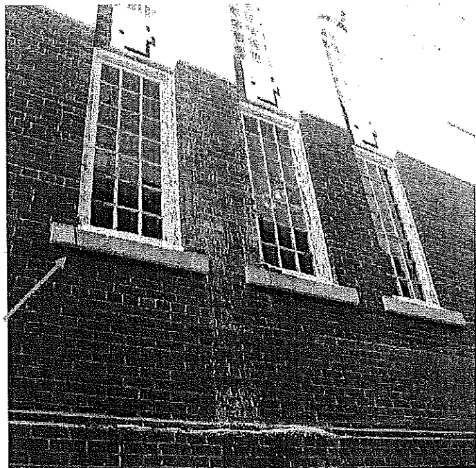
Figure 29 – South face of Chapel showing cracked Tyndall Stone sills on two windows
