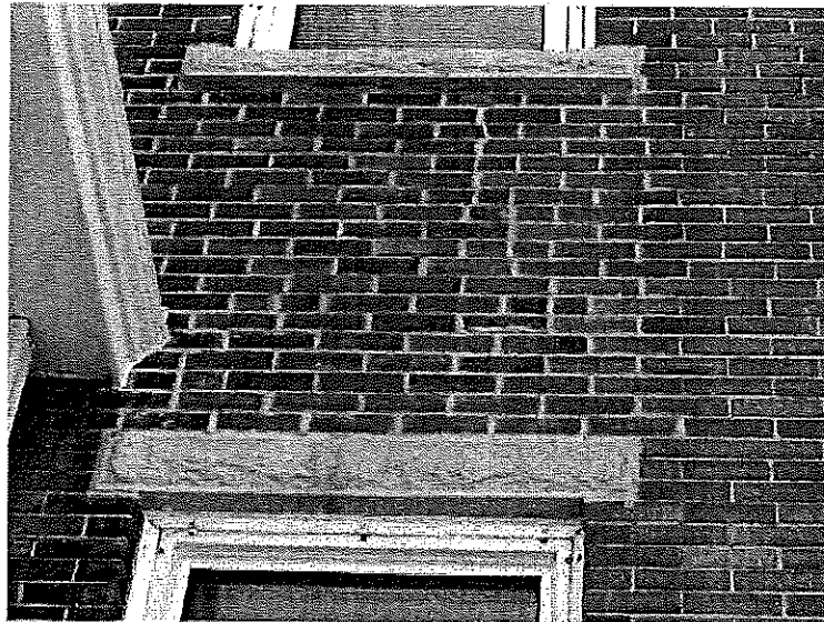
Figure 23 – East façade – note brick joints in area of replaced wall above and below windows
