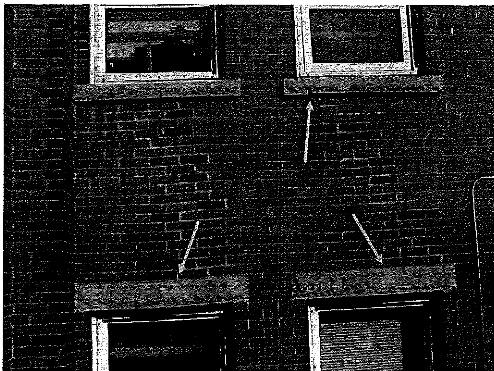
Figure 27 – Examples of cracked stone sills and lintels with evidence of previous repairs on South face beside chimney
