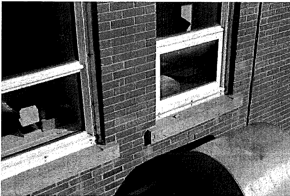
Figure 26 – Example sills with evidence of previous repairs on South face of building
