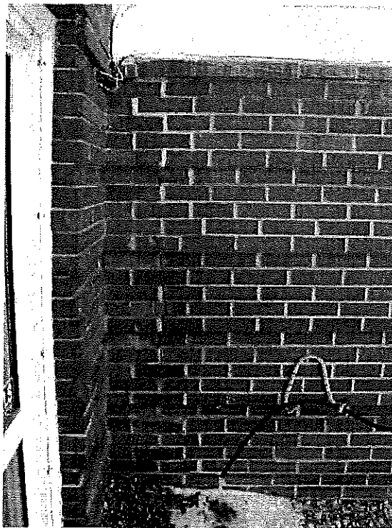
Figure 24 – Vertical crack on south side of porch on east side of building
