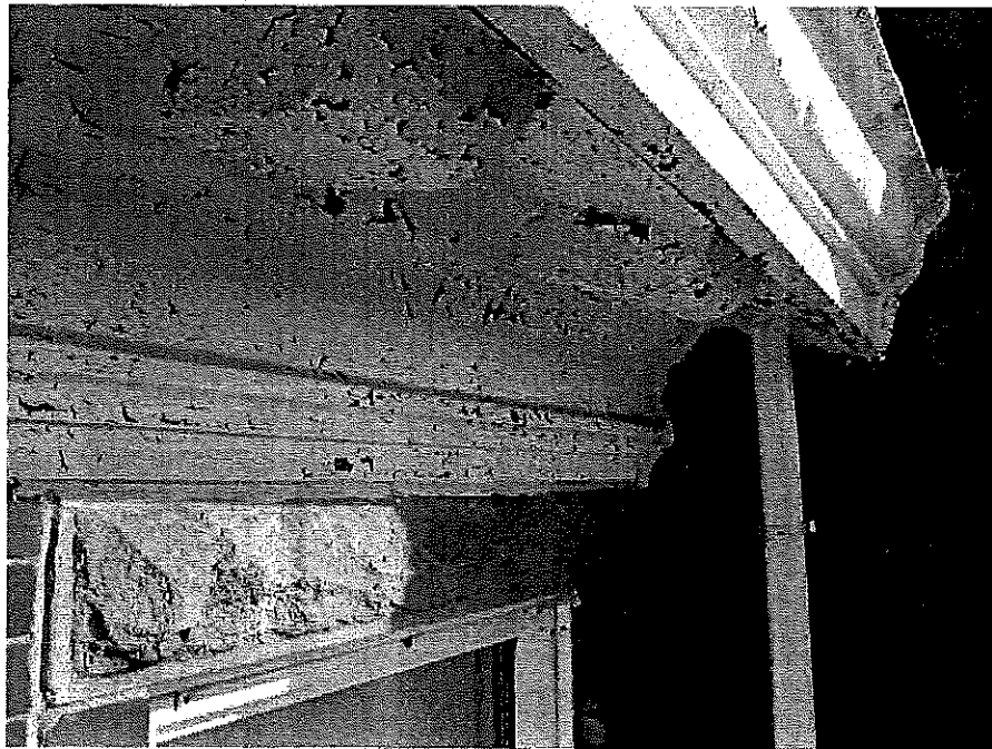
Figure 33 – profilled metal cornice on south face – noticeable deflection
