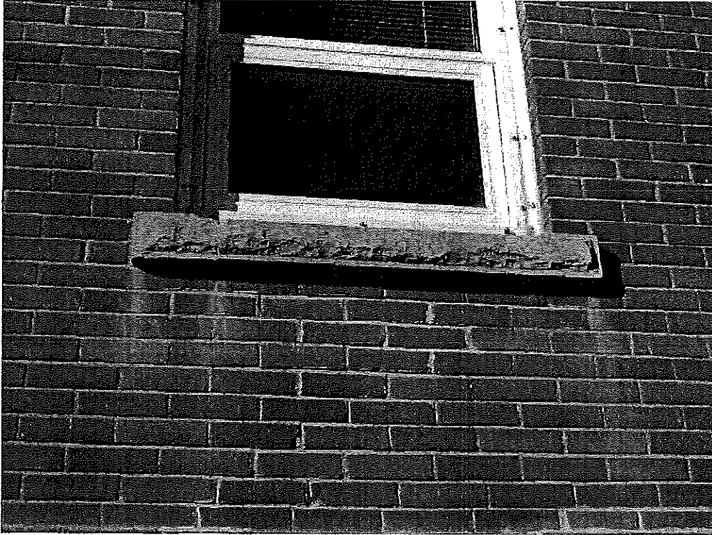
Figure 30 – Cracked limestone sill on South face of building
