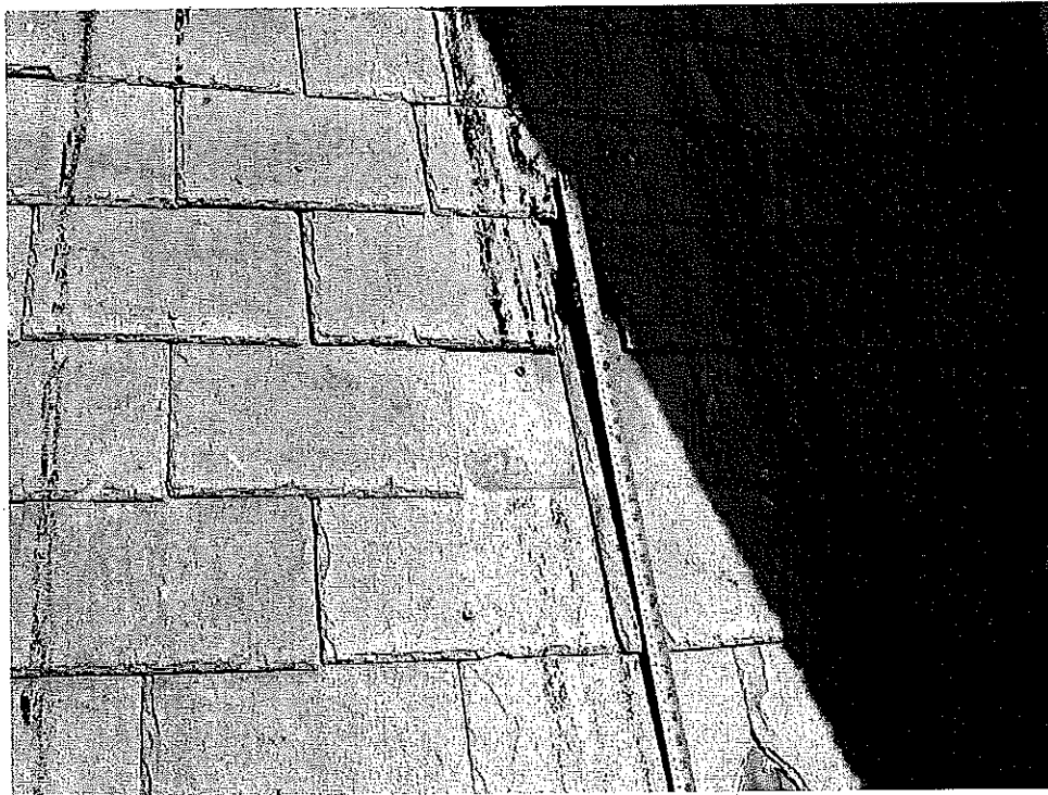
Figure 38 – South façade - missing and broken slates and fasteners through face of slates (common around building)
