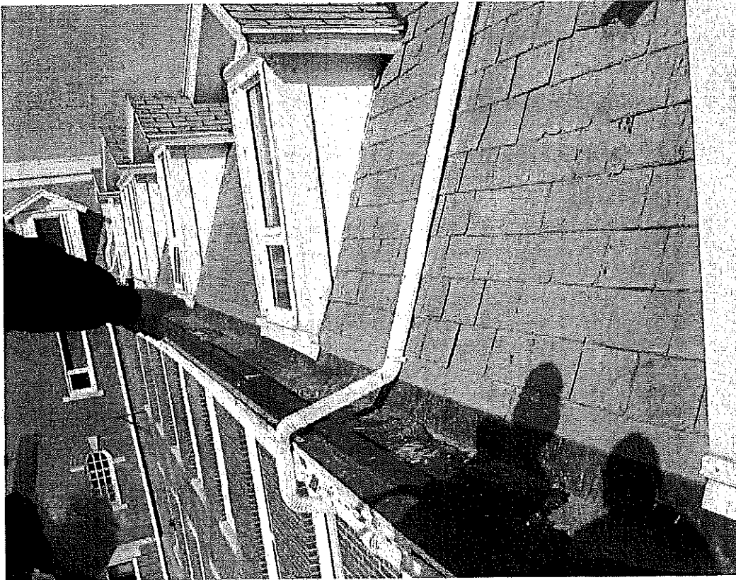
Figure 41 – South façade – plugged off roof drain location (below downspout). Also note broken, loose slates with face fastening.
