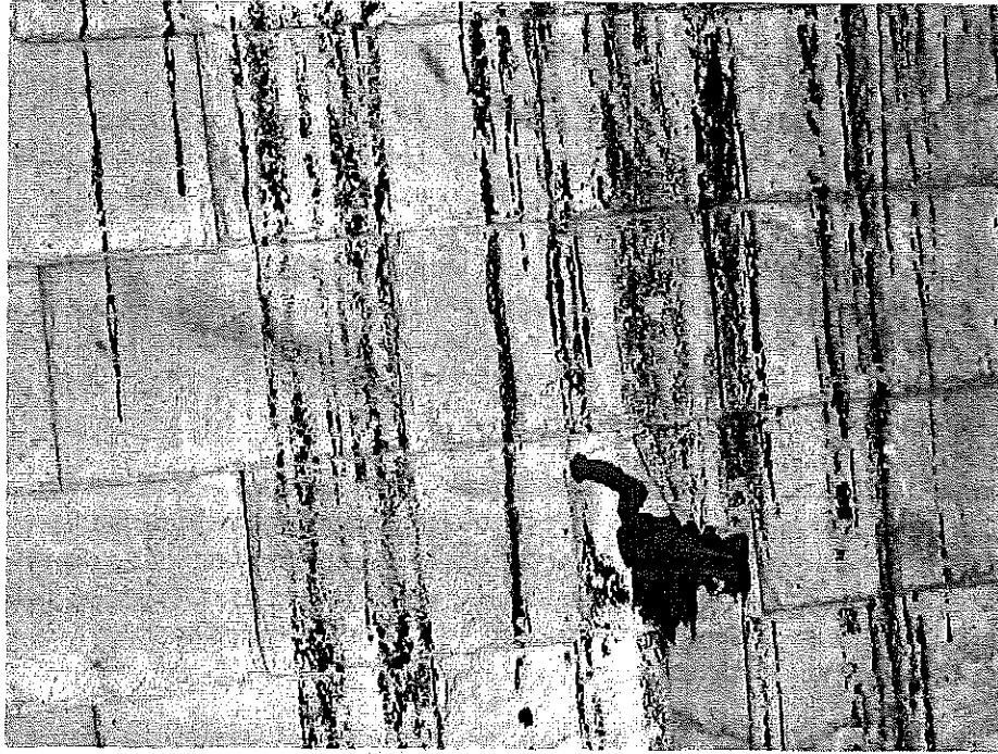
Figure 39 – South façade— asphalt or tar on slates (common around building)
