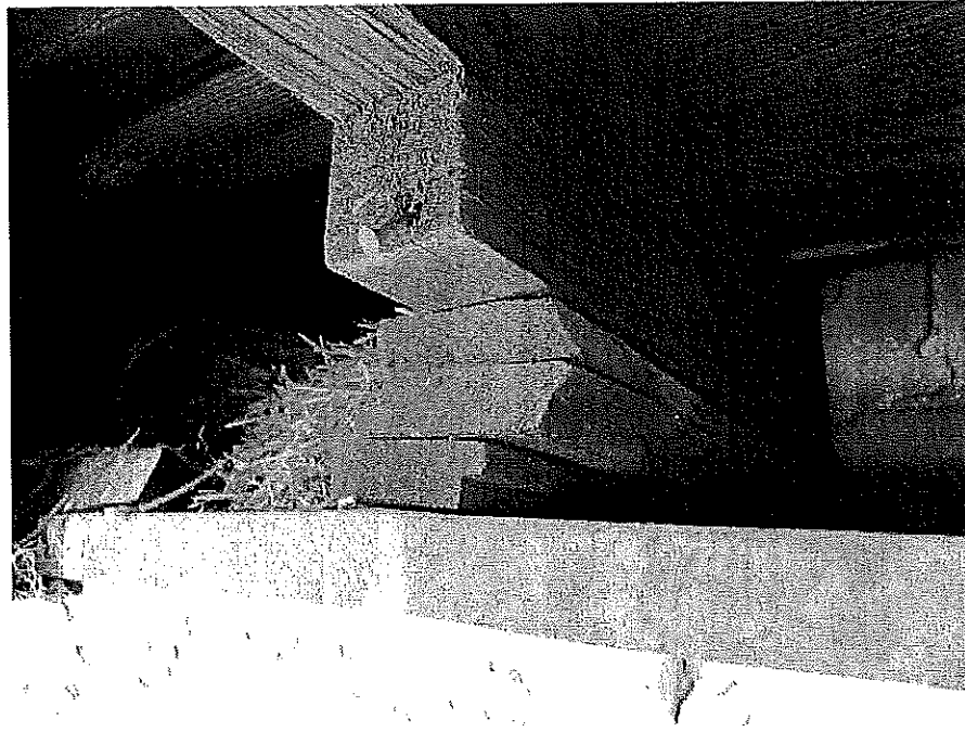
Figure 34 – showing wood framing and furring (note bird nest)
