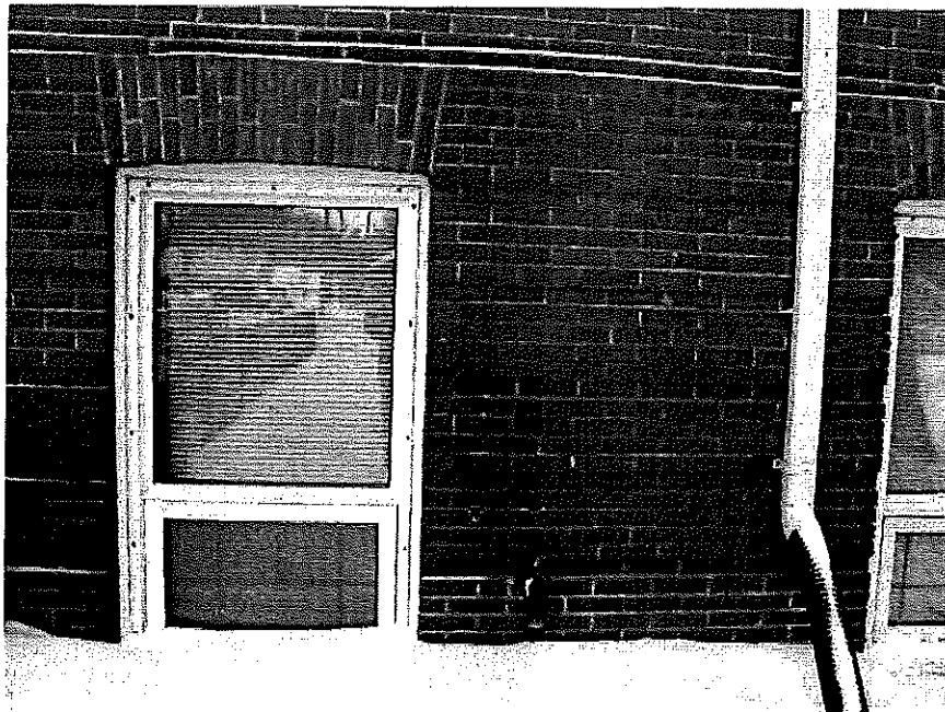
Figure 12 – Area of 1914 portion with deteriorated mortar joints (note dark staining at stepped bricks)
