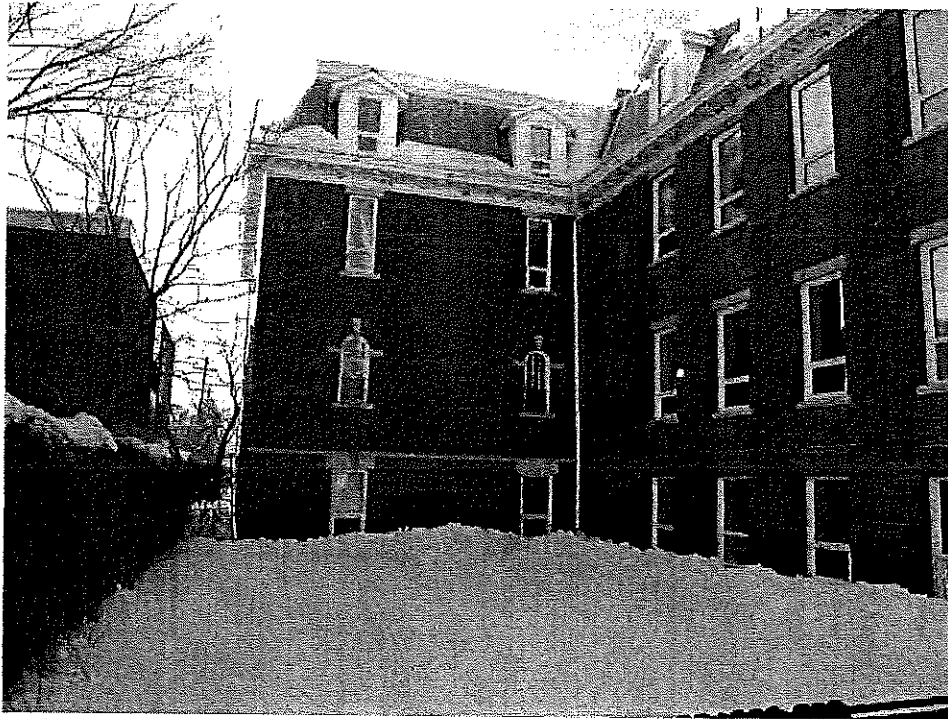
Figure 5 – South façade. 1924 portion – chapel with arched windows
