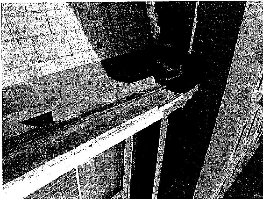
Figure 35 –top side of cornice with EPDM roofing (wet condition at chimney)
