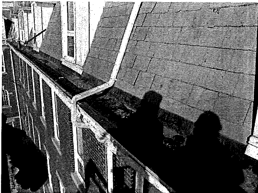
Figure 37 – top side of cornice with EPDM roofing – at least one roof drain in the cornice appear to have been closed off (red arrow).
