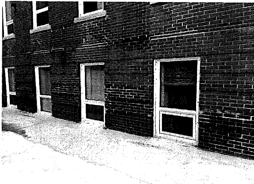
Figure 21 – South façade – note running bond above windows where original brick arches have been replaced
