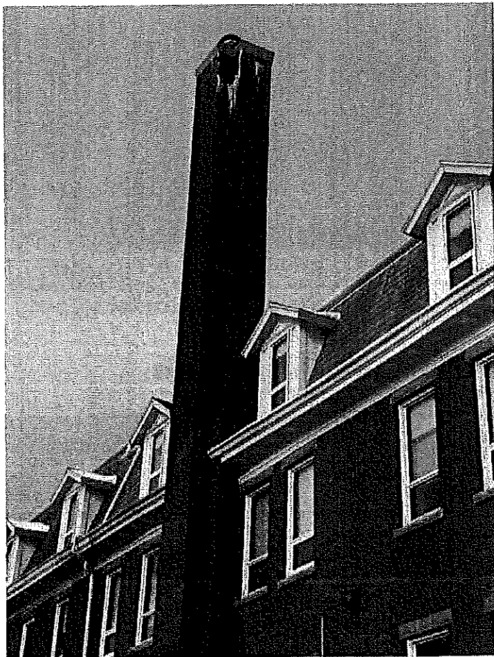
Figure 25 a) – Chimney is wet from combustion gasses seeping through flue liner.
