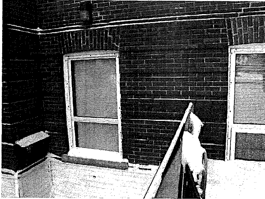
Figure 11 – Area of 1914 portion with deteriorated mortar joints
