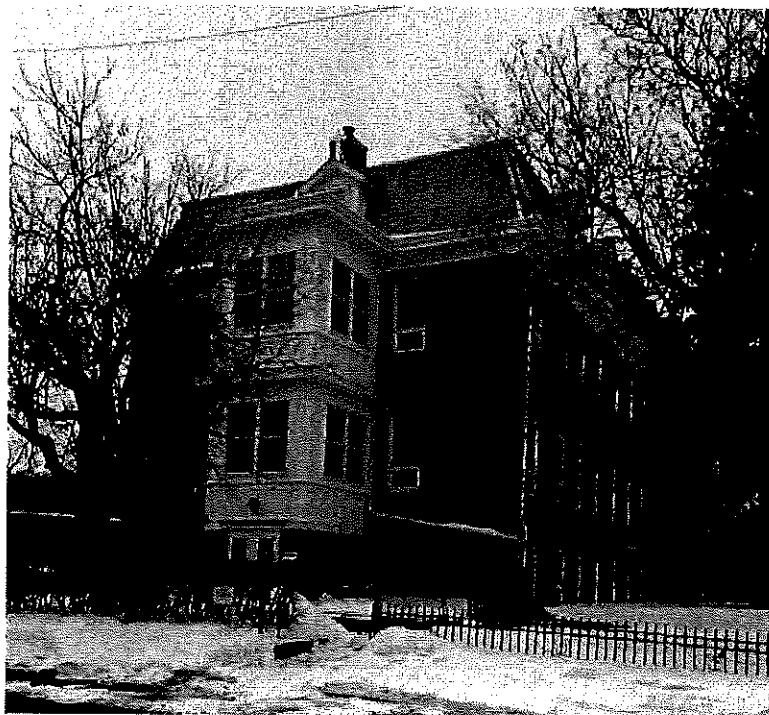
Figure 5 – East façade. 1909 portion. Showing enclosed porch at this end
