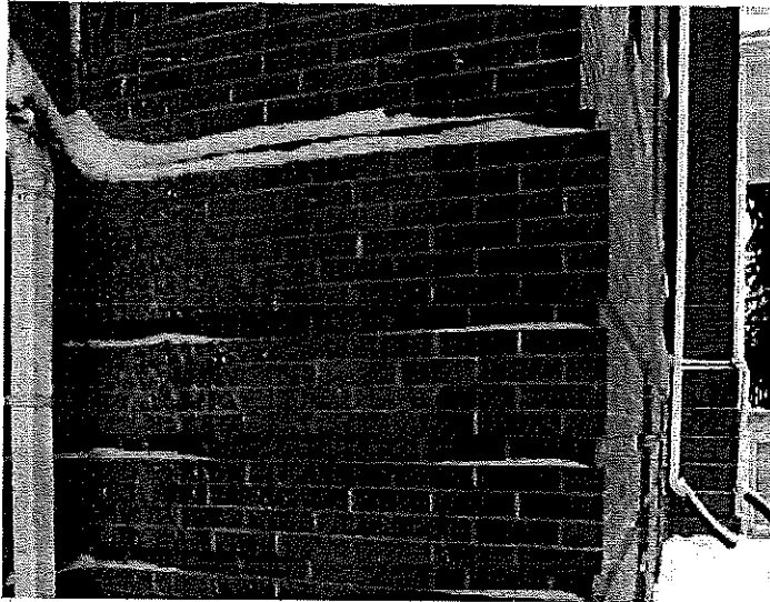
Figure 8 – double projecting brick courses at top of rustication on 1909 and 1914 portions
