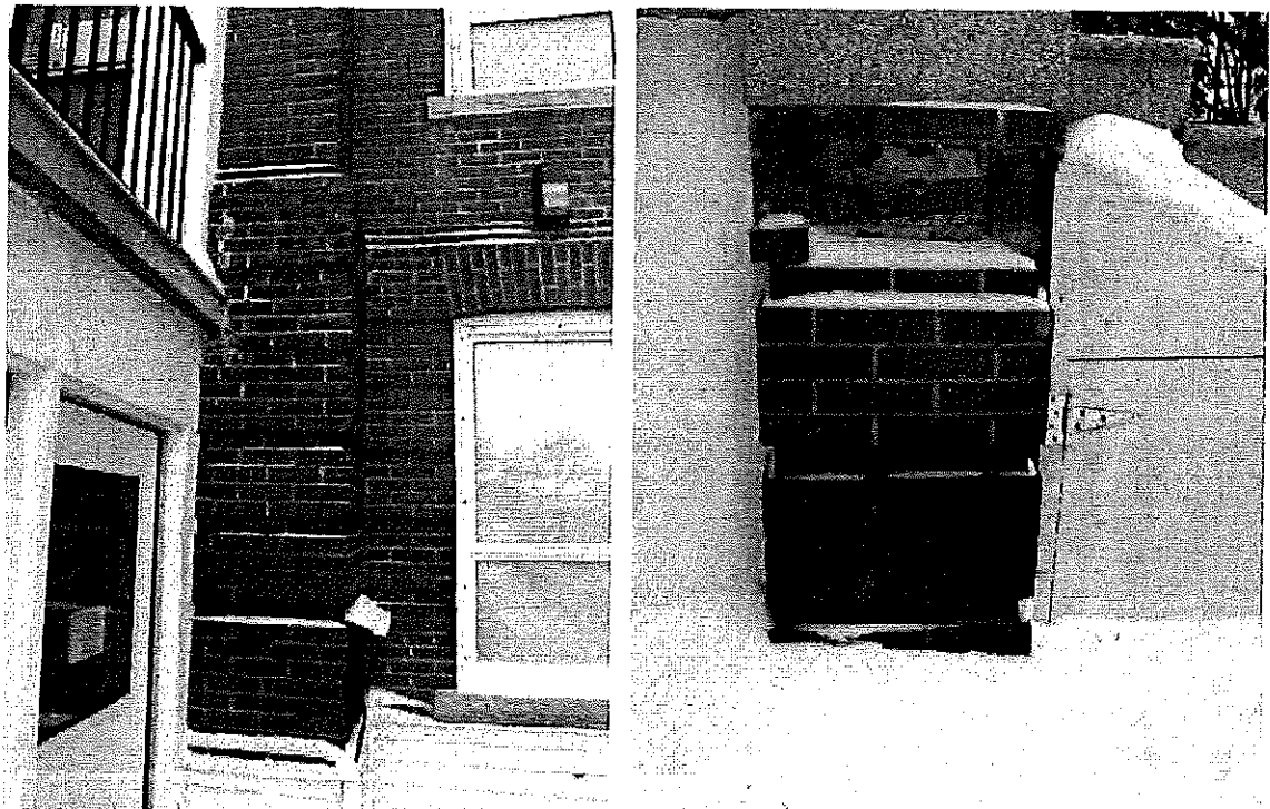
Figure 15 (left) – West side of stair – similar damage at landing both sides of main entrance Figure 16 (right) – East side of stair – bricks missing on pilaster of main entrance
