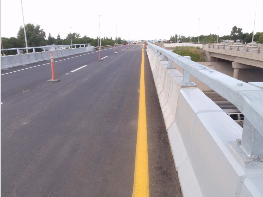
Ring Road South Bound over Dewdney Bridge Rehabilitation in 2011
