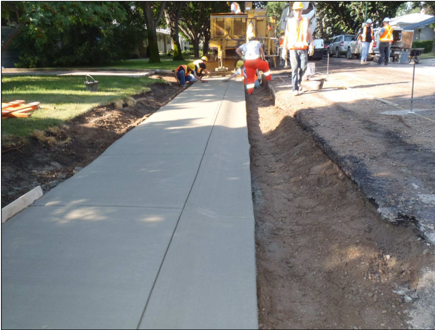
Slip Forming New Sidewalk as part of LIP Project
