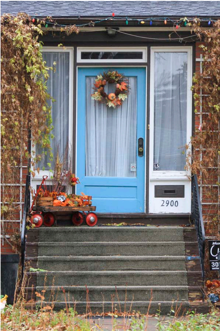
Caption: Detail of the main entryway to the verandah on the front elevation of the Hacker Residence.
