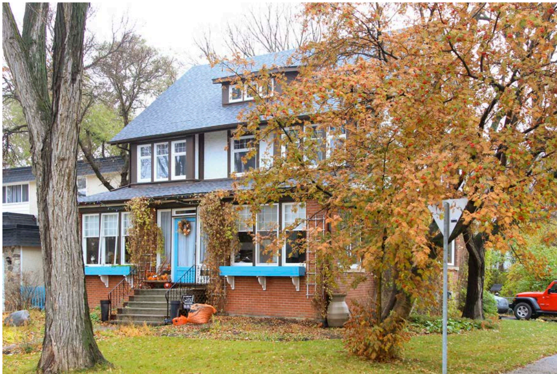
Caption: Obscured view of the front (left) and north (right) elevations of the Hacker Residence.
