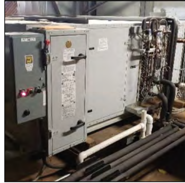
Figure 6.5.11 Fitness Area HVAC Unit
