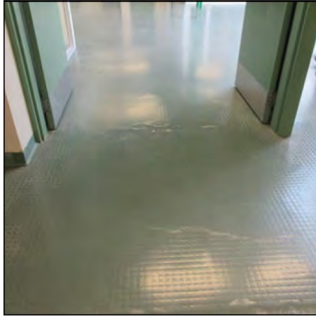
Figure 3.5.1 Entry Resilient Flooring
