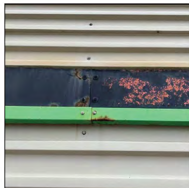
Figure 4.4.16 Corrosion at Steel Band, Fieldhouse
