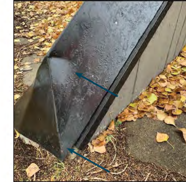
Figure 4.4.3 Corrosion and Damage, Concrete Buttresses, Steel Cap
