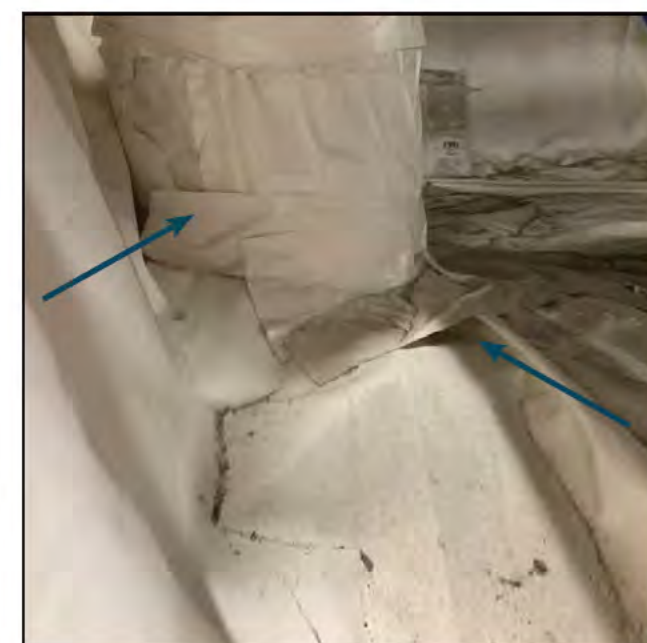
Figure 4.4.56 Debonding of Permalon Membrane, Crawspace
