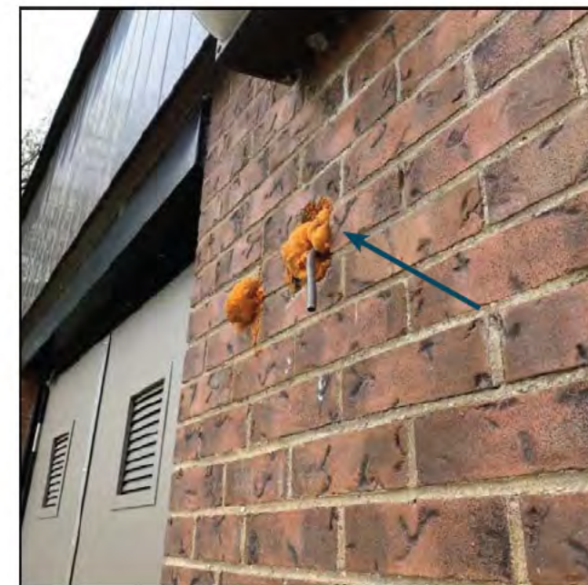
Figure 4.4.35 Spray Foam Being Used as Sealant, North Elevation
