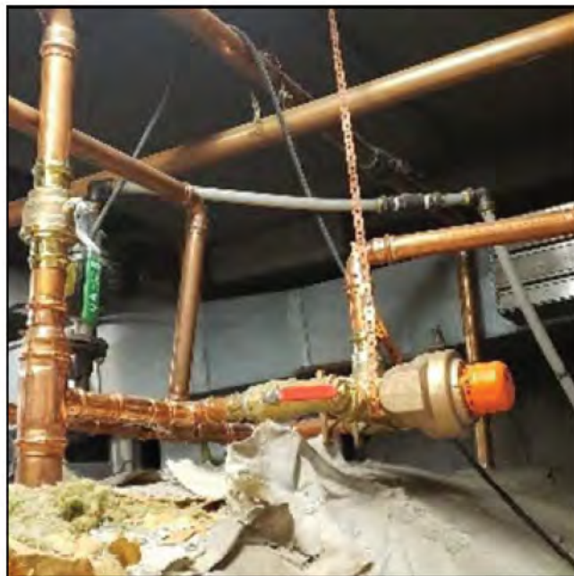
Figure 6.5.13 Domestic Hot Water Piping in Boiler Room
