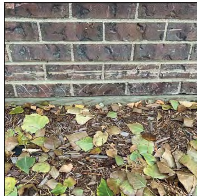
Figure 4.4.26 Wood at Base of Brick Veneer, West Elevation
