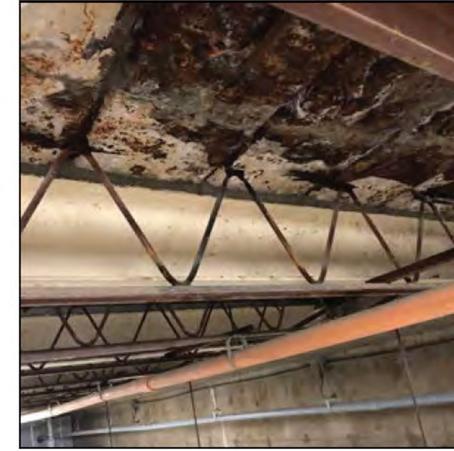
Figure 5.3.10 Corroded Steel Floor Joist
