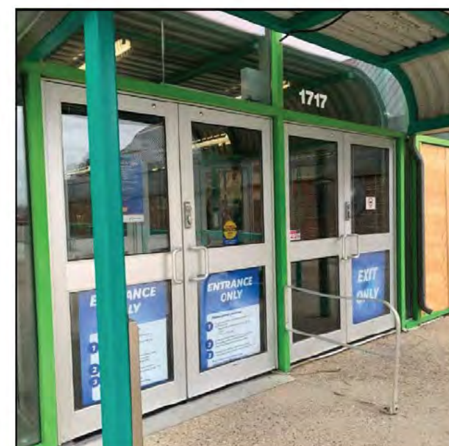
Figure 4.4.40 Main Entrance Doors, Linking Building
