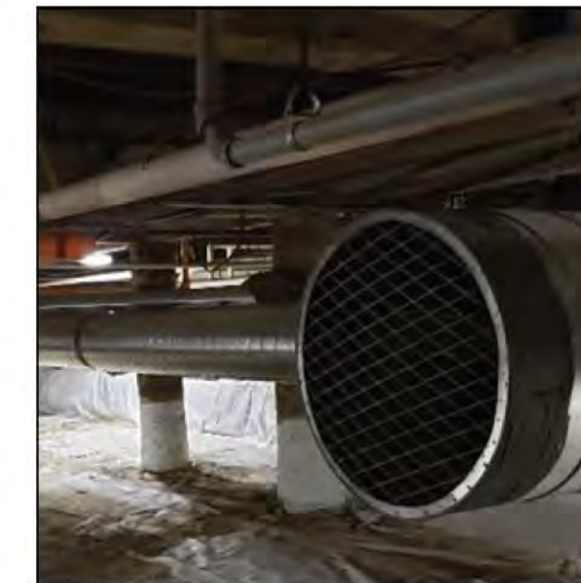
Figure 6.5.6 Crawspace Ventilation Ductwork
