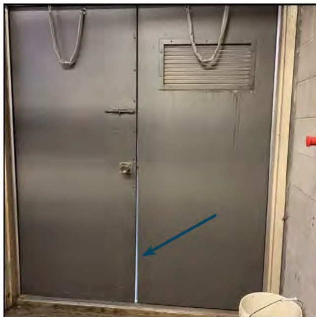
Figure 4.4.41 Gaps at Service Doors
