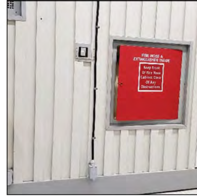
Figure 6.5.20 Firehose / Extinguisher Cabinets
