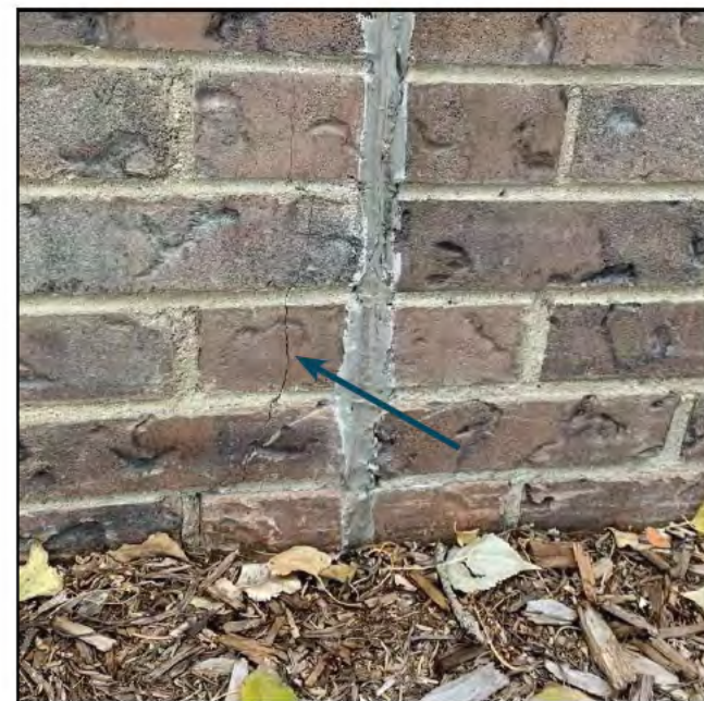
Figure 4.4.27 Cracking at Brick Veneer Near Vertical Control Joint
