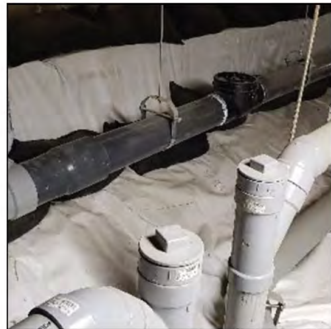
Figure 6.5.14 Crawspace Sanitary Piping
