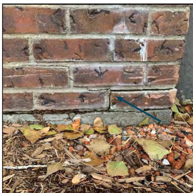
Figure 4.4.29 Deteriorating Mortar Around Bricks
