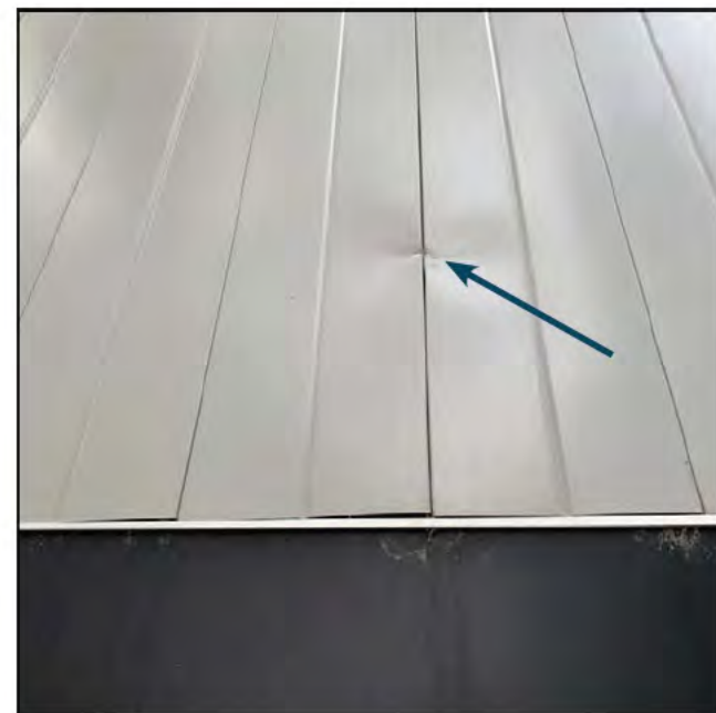
Figure 4.4.12 Damaged Metal Cladding, West Wall
