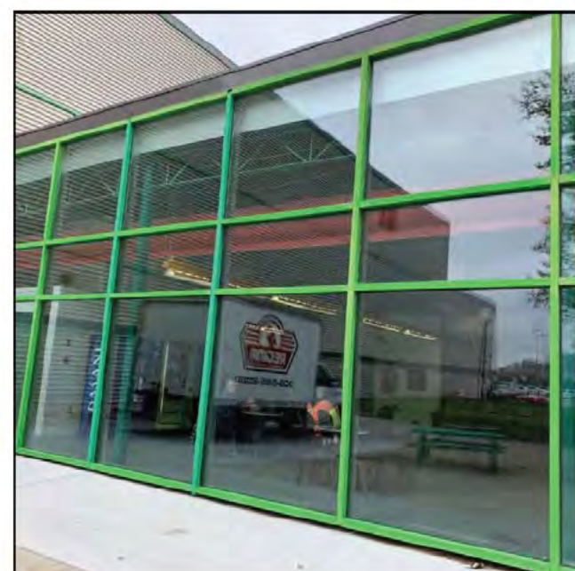
Figure 4.4.32 Curtain Wall Assembly, Linking Building
