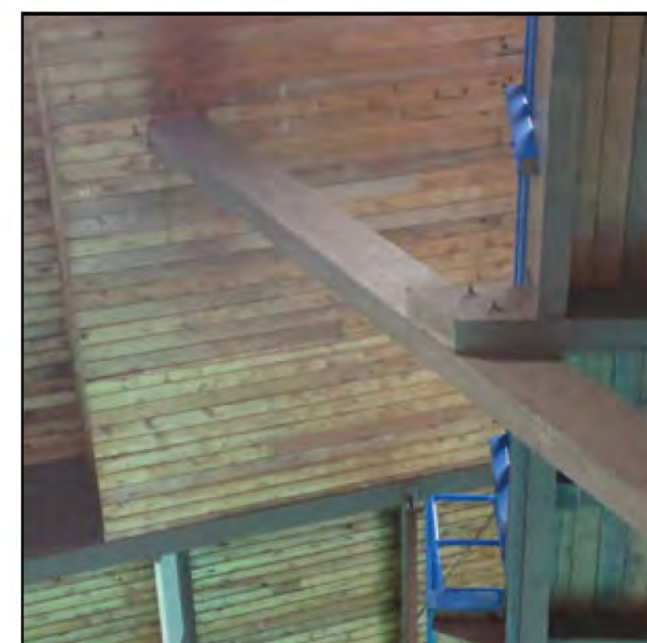
Figure 3.5.30 Diving Tower Ceiling
