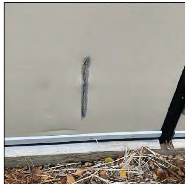
Figure 4.4.42 Damage to Door Exteriors, Fieldhouse
