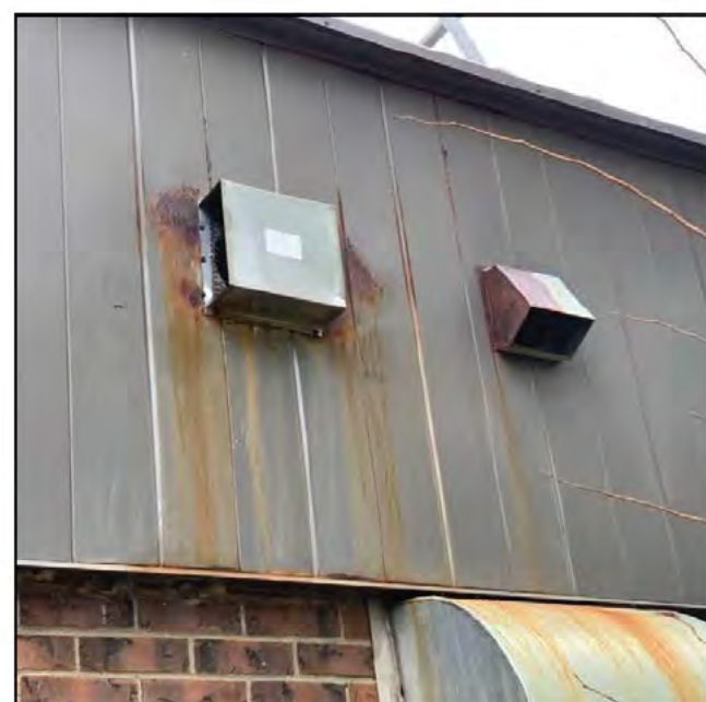
Figure 4.4.14 Corrosion of Metal Cladding, North Elevation
