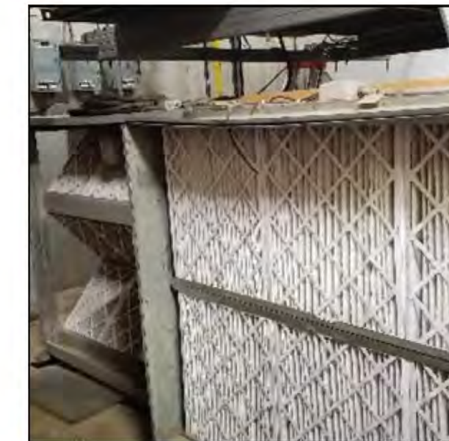
Figure 6.5.8 Pool Area Make-Up Air Units Mua-2 and Mua-3
