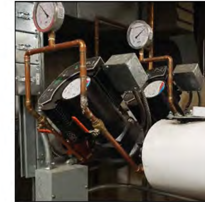
Figure 6.5.3 Secondary Heating Pump
