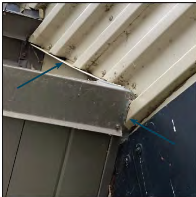
Figure 4.4.25 Interface with Gaps and Poor Sealants, West Elevation
