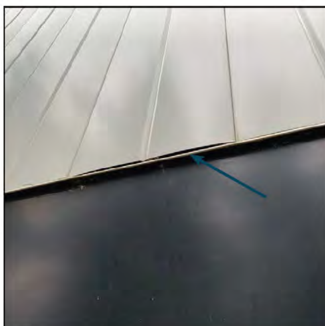
Figure 4.4.13 Separation of Metal Cladding From Wall
