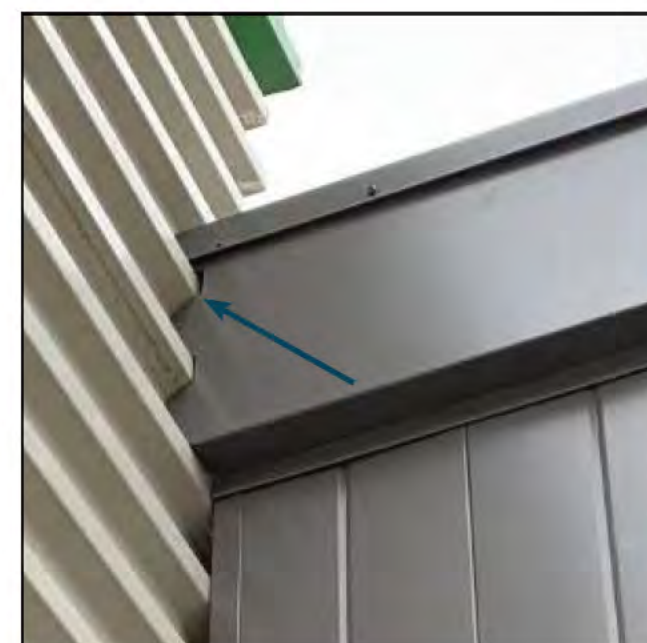
Figure 4.4.22 Gaps at Cladding Interface, East Elevation
