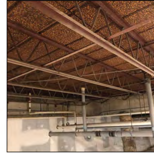
Figure 5.3.11 Underside of Main Floor Corrosion
