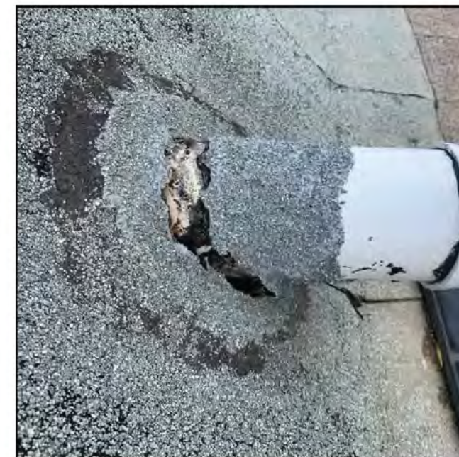
Figure 4.4.52 Splitting of Roofing Membrane at Penetration, South Roof
