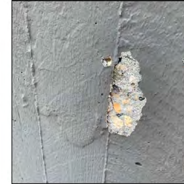
Figure 4.4.2 Spalling, Concrete Buttress
