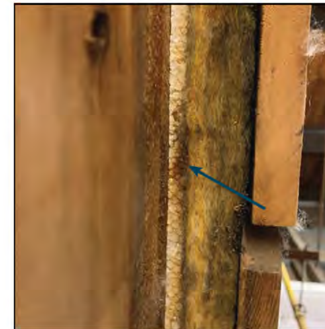
Figure 4.4.5 Water Staining at Interior Finish, West Wall, First Penthouse Level Above Fitness Center 2
