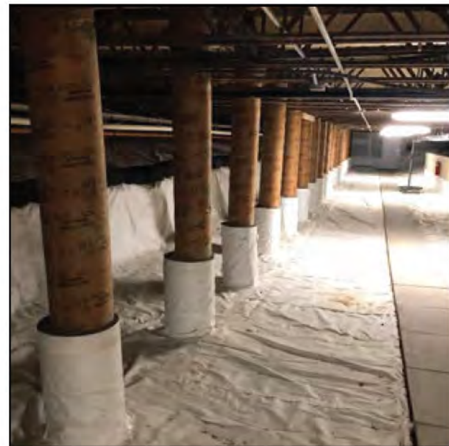
Figure 5.3.6 Main Floor Reinforcing Foundations
