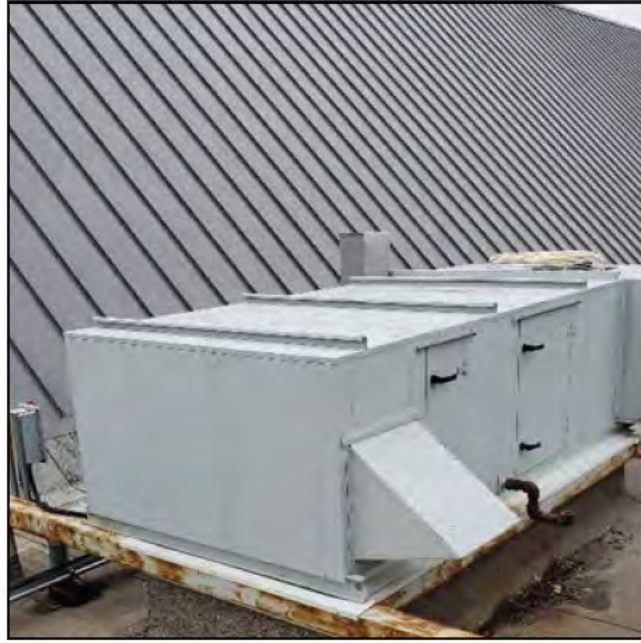
Figure 6.5.9 Roof-Top Unit Rtu-1
