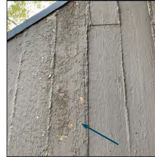
Figure 4.4.1 Peeling Paint, Concrete Buttress
