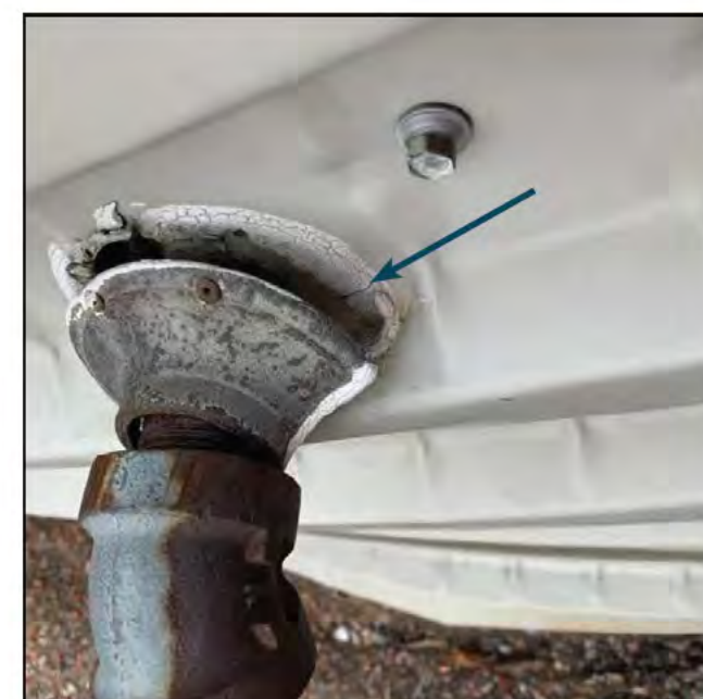
Figure 4.4.38 Sealant at Penetration, Fieldhouse
