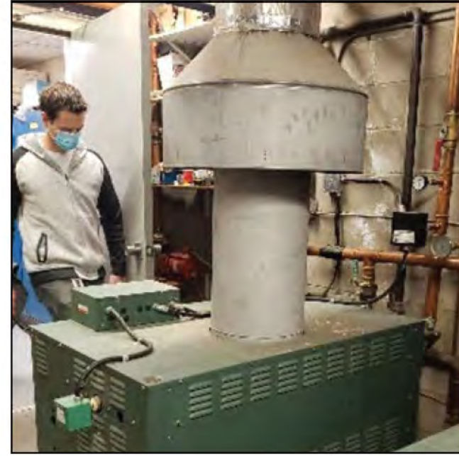
Figure 6.5.12 Domestic Hot Water Boilers
