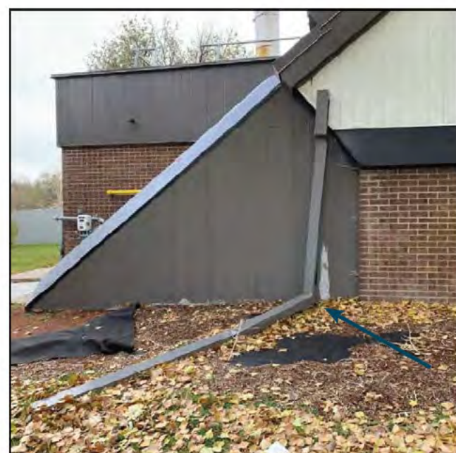
Figure 4.4.46 Damaged Downspout, West Elevation
