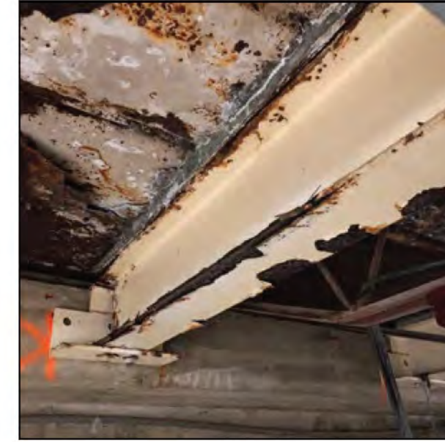
Figure 5.3.9 Steel Reinforcing Beam
