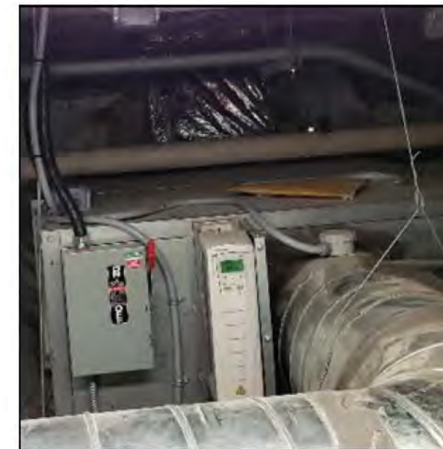
Figure 6.5.5 Crawspace Make-Up Air Ventilation Unit
