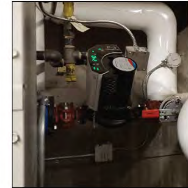
Figure 6.5.2 Boiler Circulation Pump
