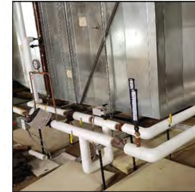
Figure 6.5.4 Freeze-Damaged Pool Ventilation Reheat Coil
