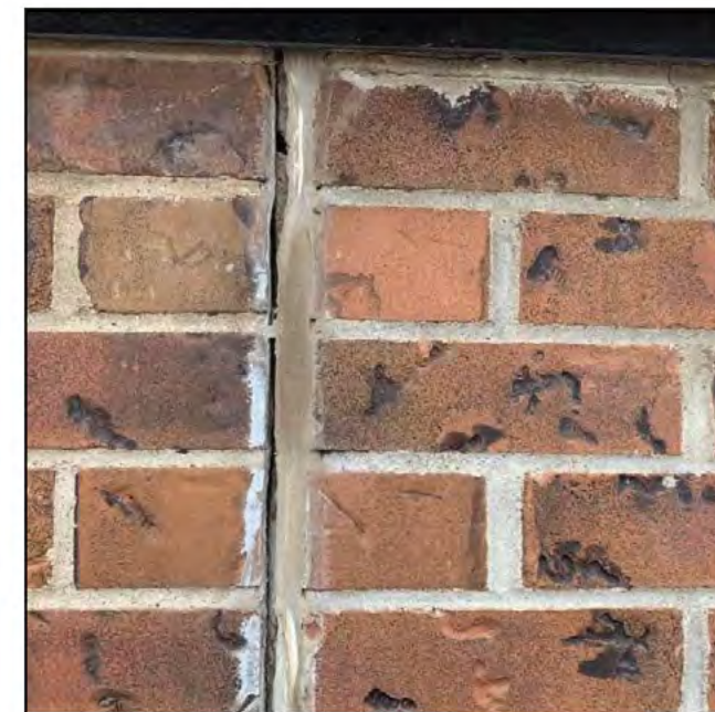
Figure 4.4.36 Split Sealant at Brick Control Joint
