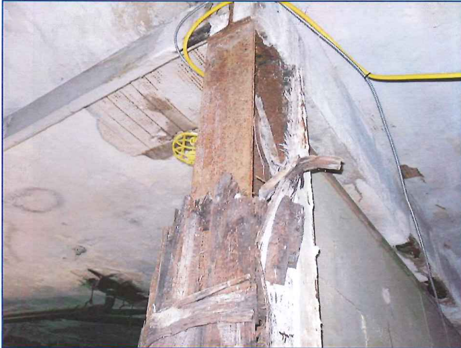
Photo 3 – Exposed Steel Column Supporting Second Floor
