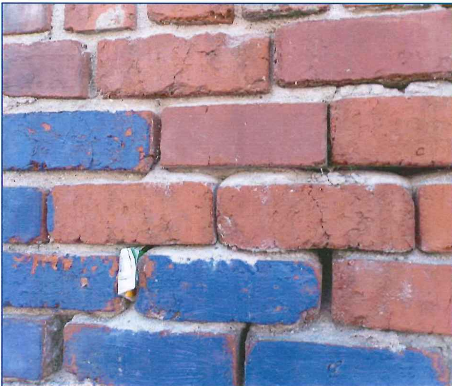
Photo 20 – North Wall Mortar Joints
