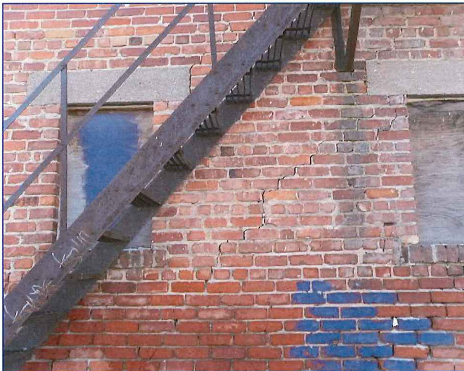
Photo 18 –North Wall Masonry
