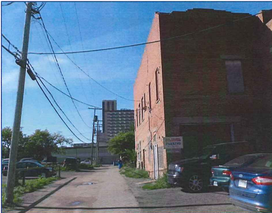
Photo 16 – Looking Along East Wall (From North)
