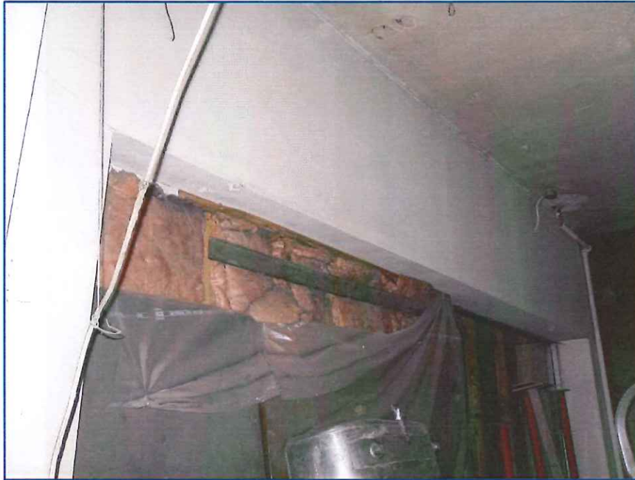
Photo 7 – Hoarding at Former Store Front (1)
