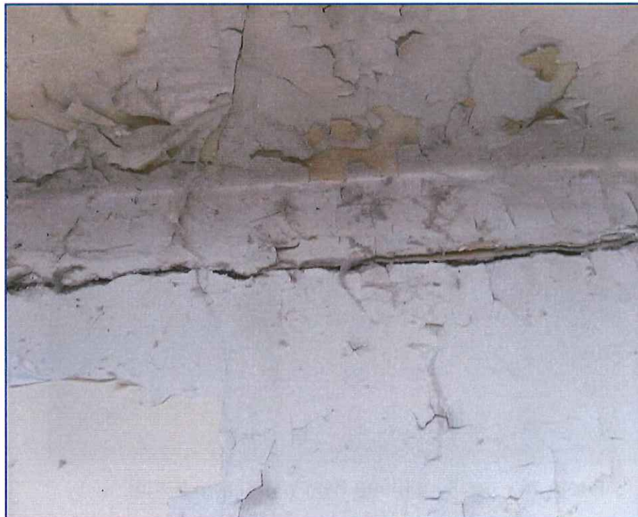
Photo 14 – Second Floor Interior Paint Finish
