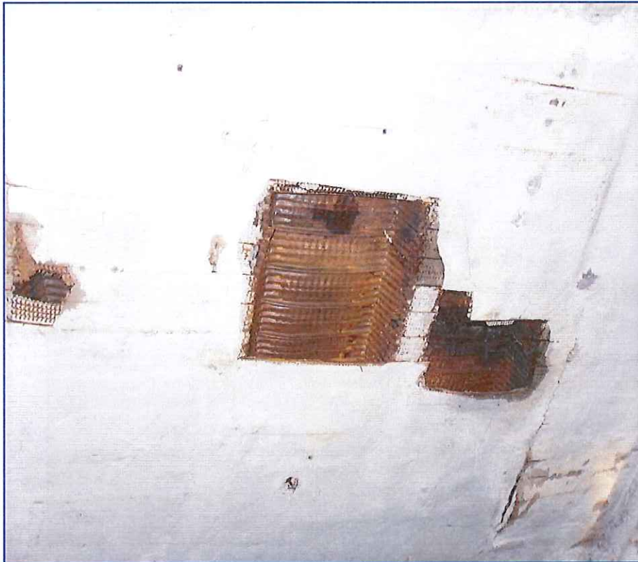
Photo 2 – Exposed Metal Pan from Second Floor Concrete Structure
