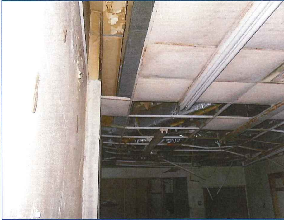
Photo 9 – T-Bar Ceiling on North Side of Main Floor
