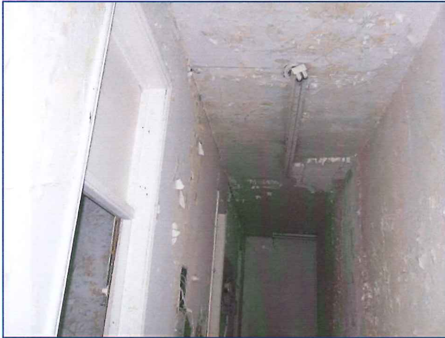
Photo 11 – Second Floor Corridor Finishes
