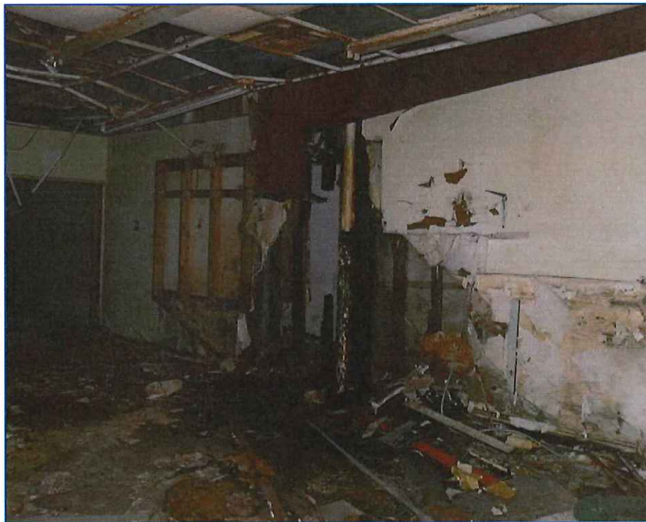
Photo 10 – Wall and Ceiling along North Side of Main Floor
