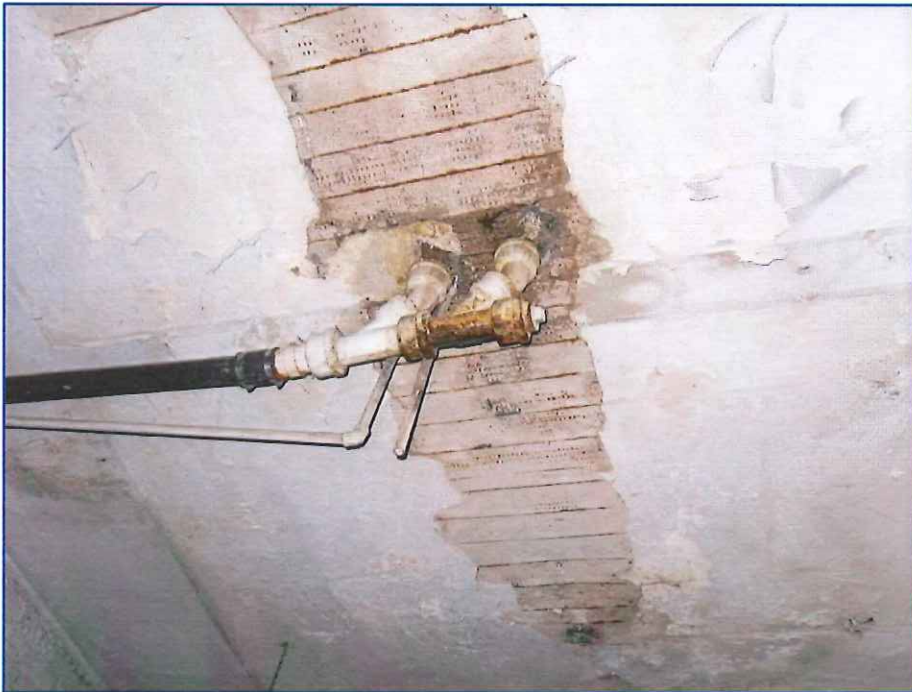
Photo 4 – Exposed Second Floor Deck at Mechanical Penetration
