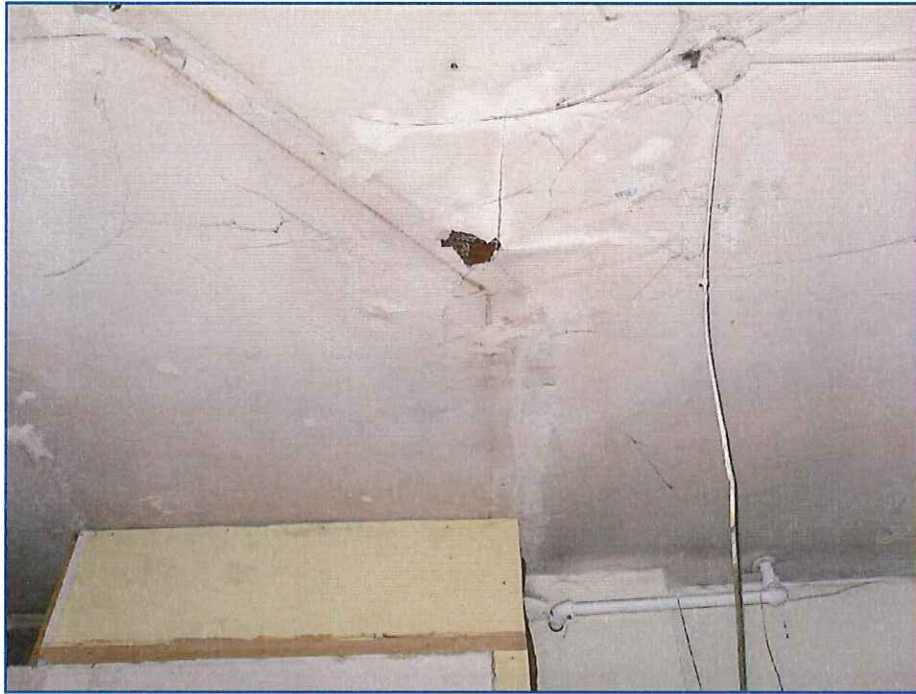
Photo 5 – Main Floor Ceiling
