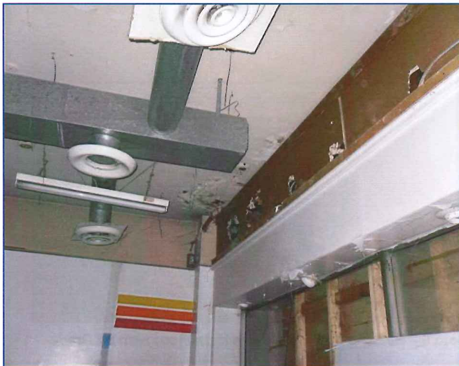
Photo 8 – Hoarding at Former Store Front (2)
