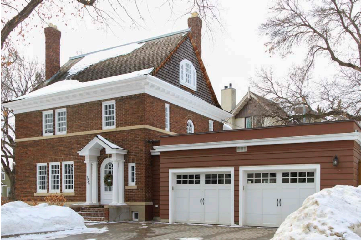
Caption: View of the front (left) and north (centre) elevations of the Willoughby Residence with attached garage on the right.
