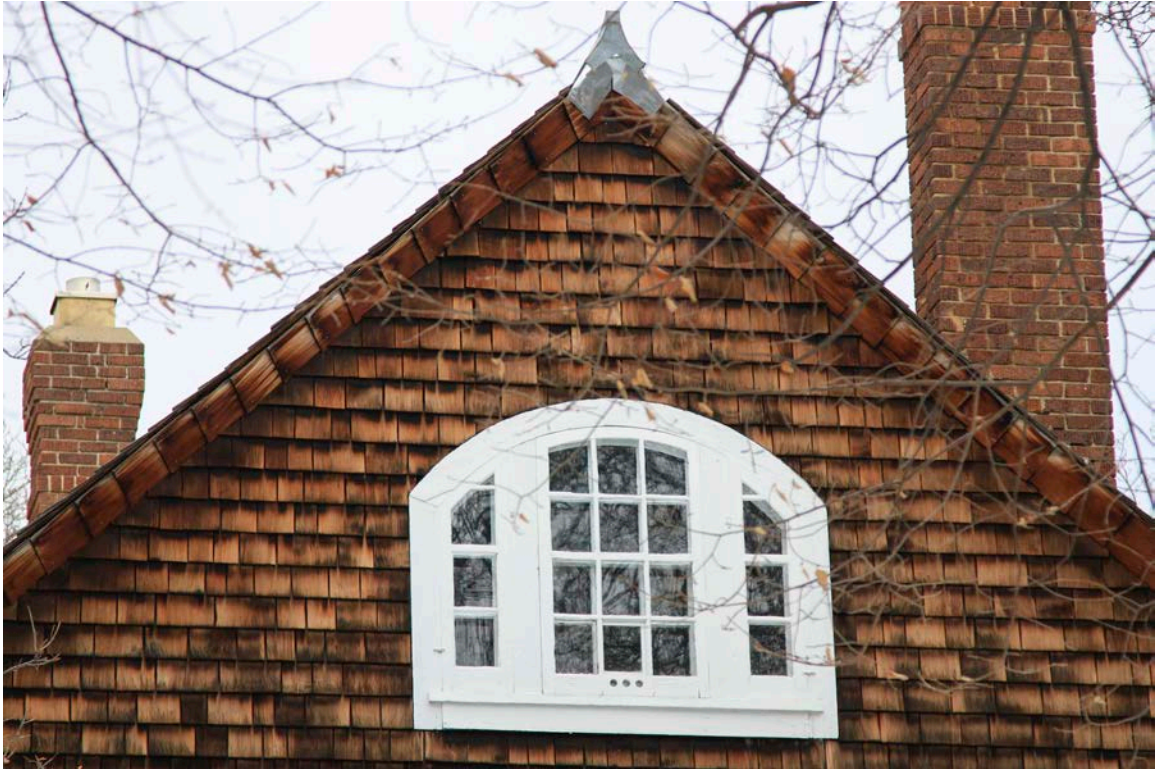
Caption: Detail of the wood shingle cladding in the Willoughby Residence’s south elevation gable; segmental arch window assembly; and metal ridge cap
