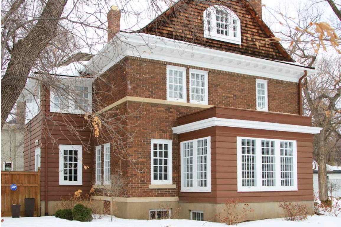
Caption: Partial view of the rear (left) and south (right) elevations of the Willoughby Residence.
