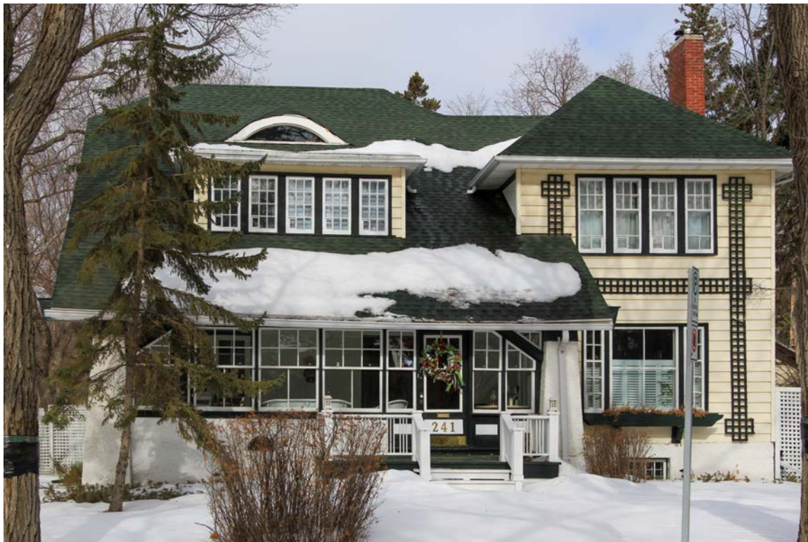
Caption: View of front elevation of the Menzies Residence.
