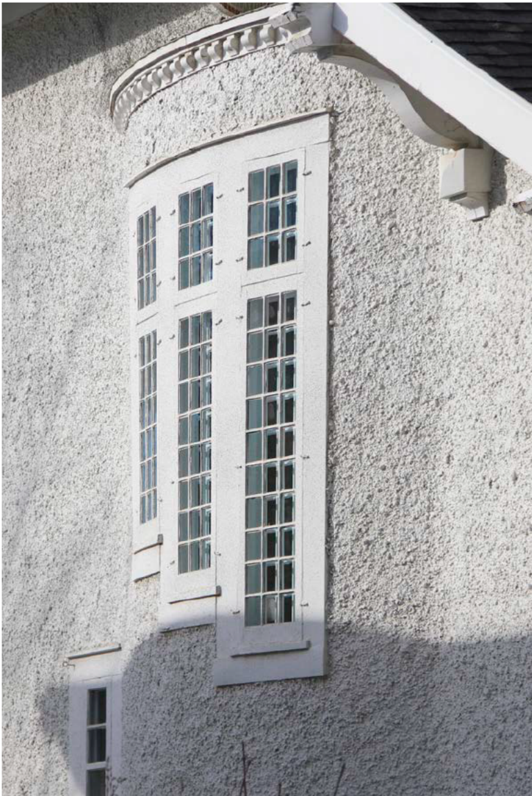
Caption: Detail of the bow window on the south elevation, presumably enclosing a staircase on the interior.
