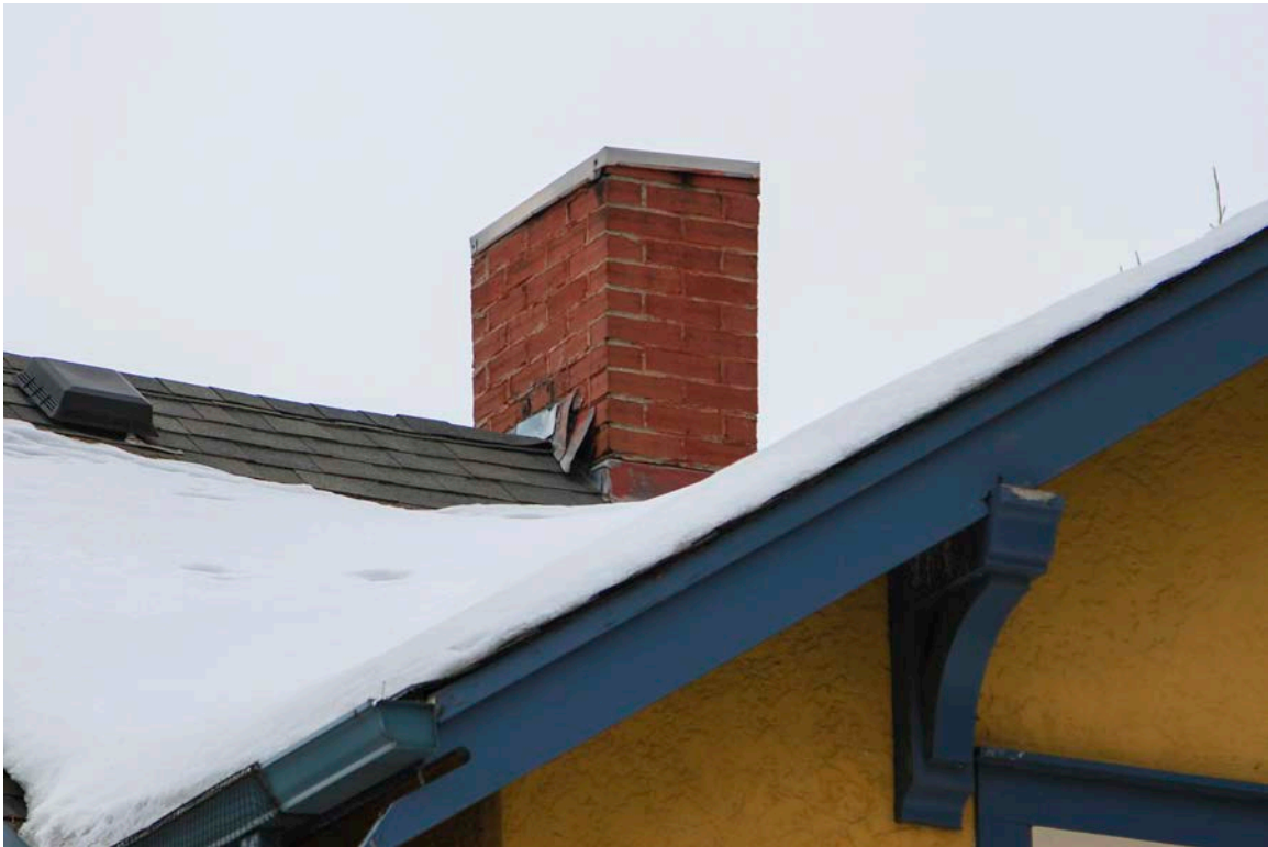
Caption: Detail of the centrally-located internal red brick chimney stack on the Cassidy Residence.
