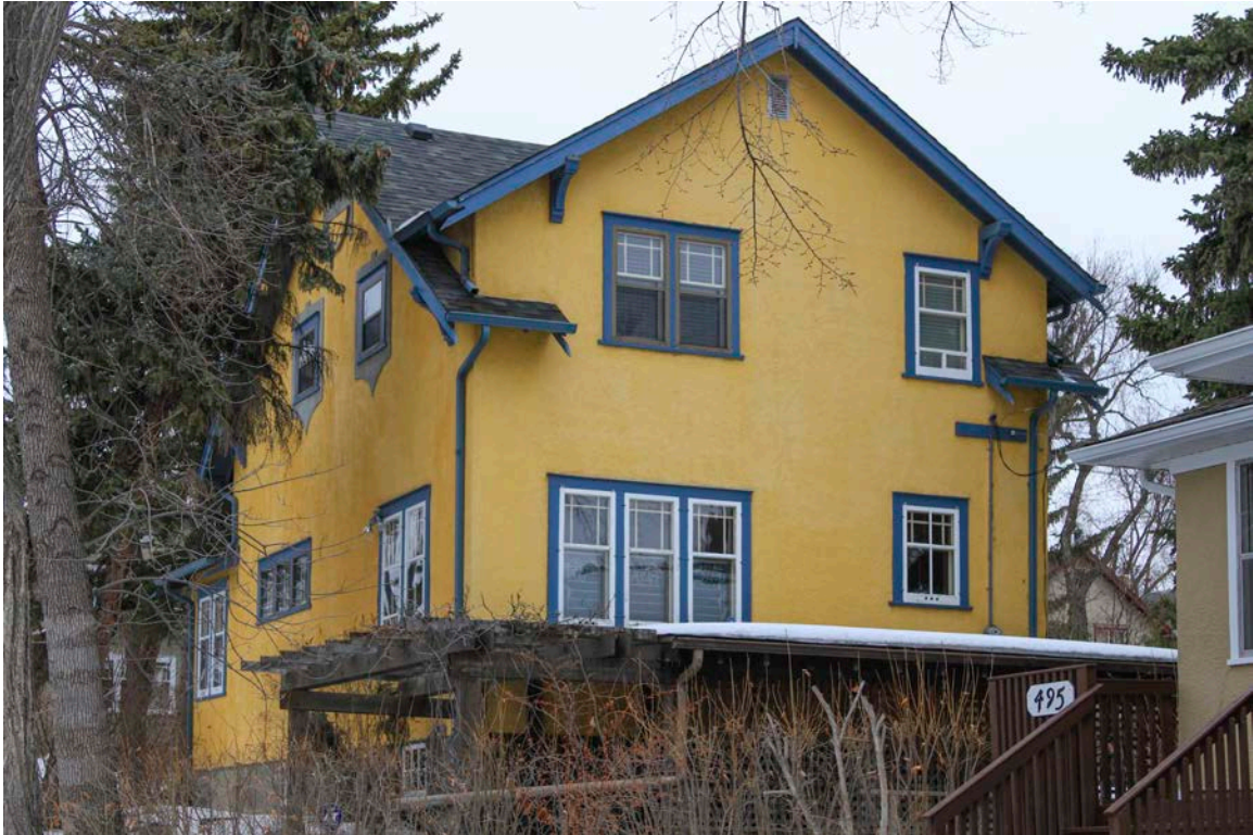
Caption: View of the rear (centre) and west (left) elevations of the Cassidy Residence.
