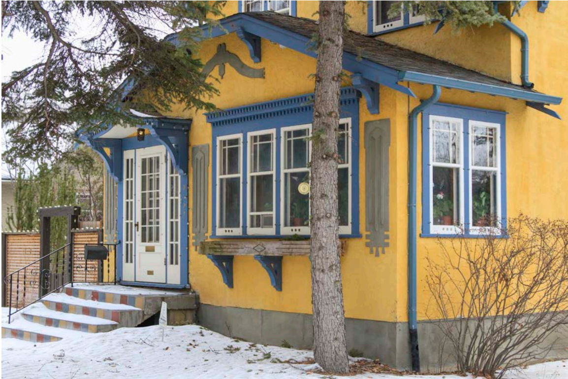
Caption: Detail of the verandah-like one-storey gable projection, with jerkinhead, on the front elevation of the Cassidy Residence.
