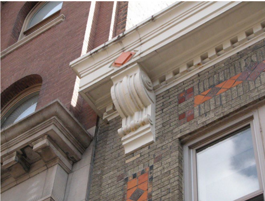
Original pressed tin rooftop cornice and grey brick with decorative tile on second floor, 2010 (City of Regina)
