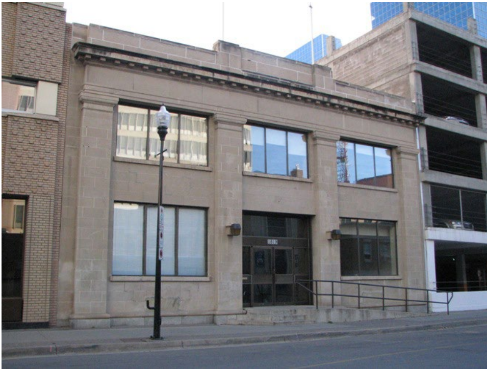
Front façade with three bays and central entry, 2010 (City of Regina)
