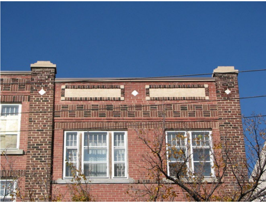
Decorative brick work on parapet with parged panels with brick surround, 2010 (City of Regina)
