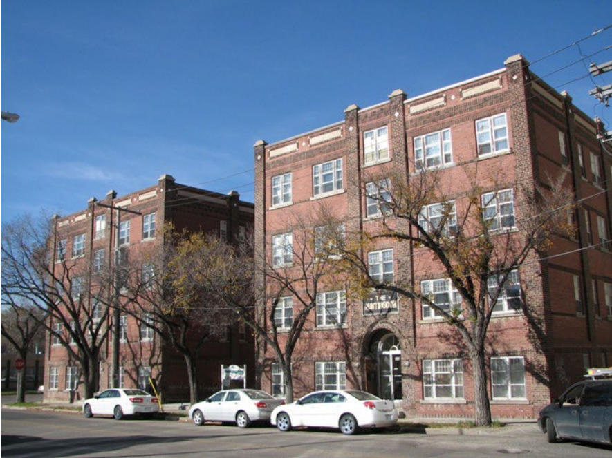
Front façade of building showing variegated brick exterior and multi-assembly windows, 2010 (City of Regina)
