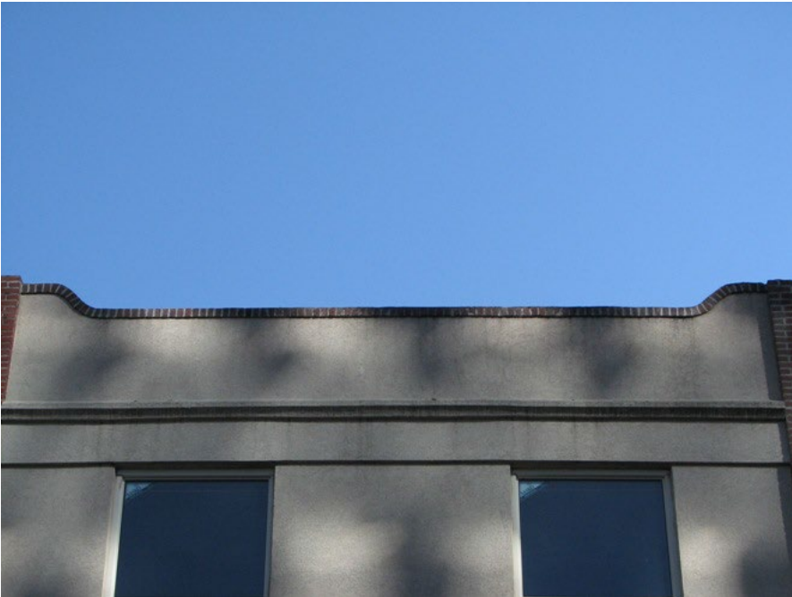
Parapet with brick cap and later added parging, 2010 (City of Regina).
