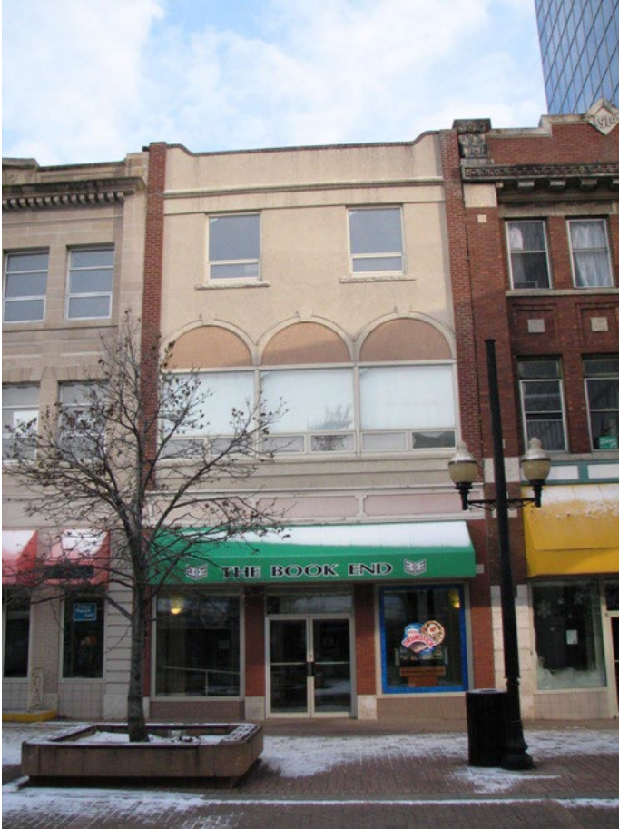
Front façade of block with ground floor “restored” in 1990s, 2010 (City of Regina)
