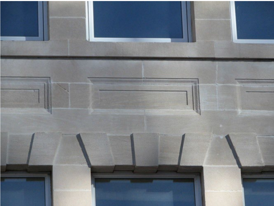
Stone voissours, window surrounds, and sills, with recessed panels between floors, 2010 (City of Regina)
